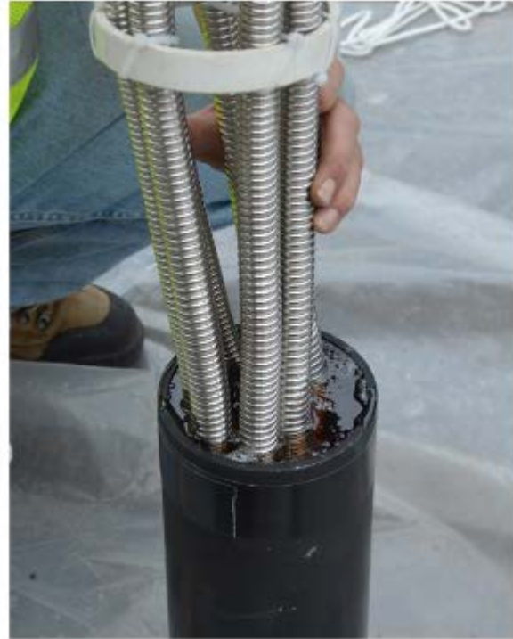
Figure 9. Tubing Preparation (left) tubing with spacers (right) epoxying the tubing
