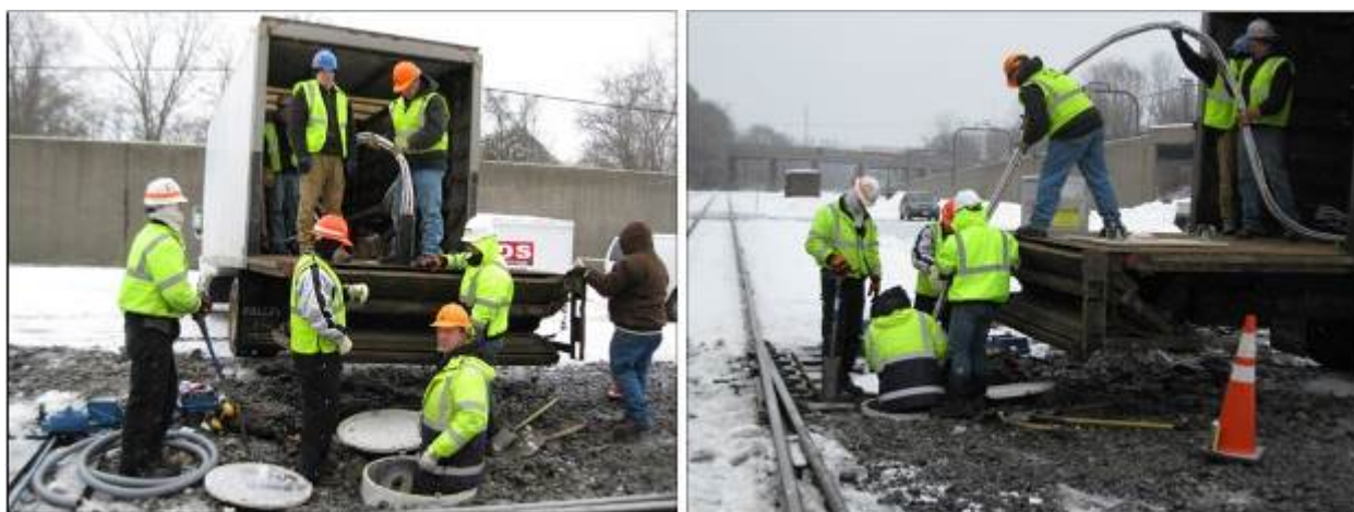
Figure 22. Installing Refrigerant Tubing into Well 2
