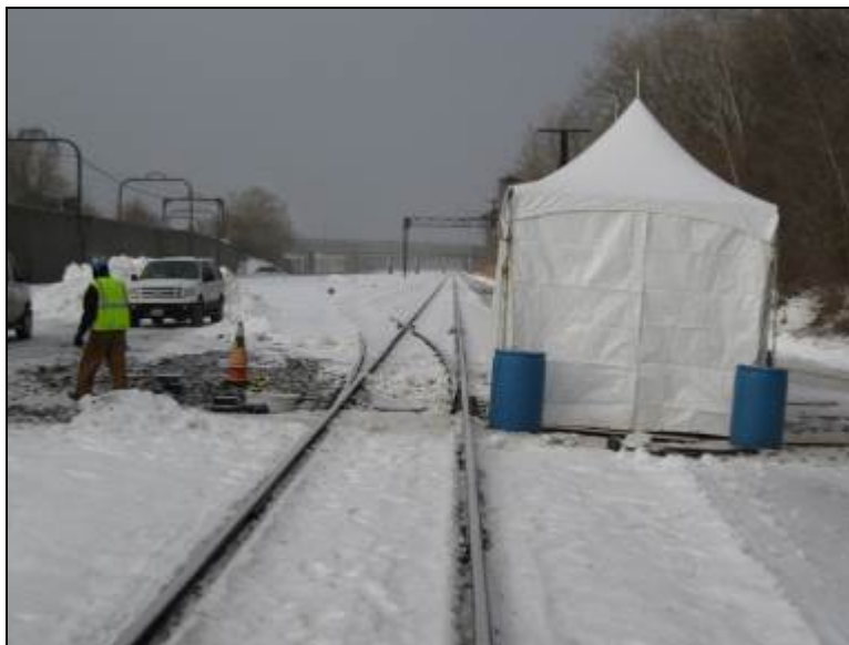
Figure 21. Phase 2 Installation of Geothermal Switch Heater
