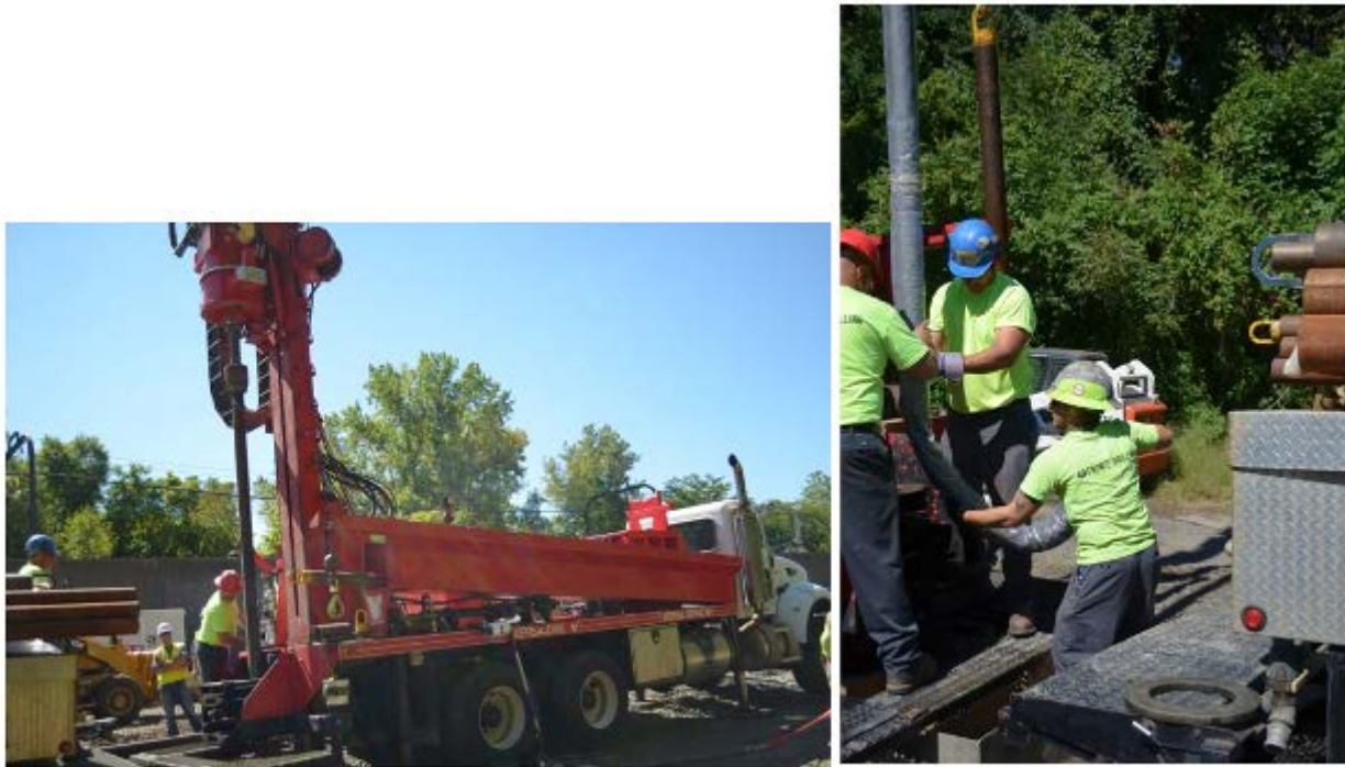
Figure 5. Drilling and Sampling Well 1
