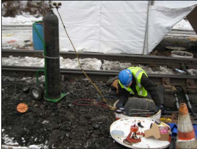
Figure 26. Purging the Systems with Nitrogen
