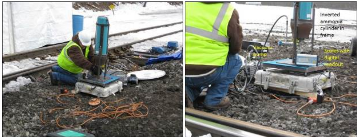
Figure 27. Charging the Heating Systems with Ammonia
