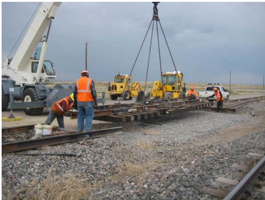
Figure 9. Test prototype crossing diamond installation
