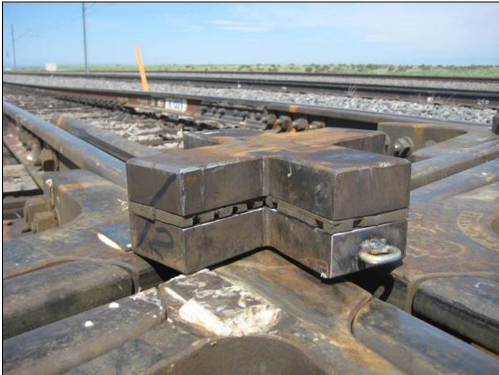
Figure 19. The steel flangeway spacer tile was cut in half and \frac{1}{4} in of material was milled from each half to accommodate a layer of the \frac{1}{2} -in Nortrak pad material
