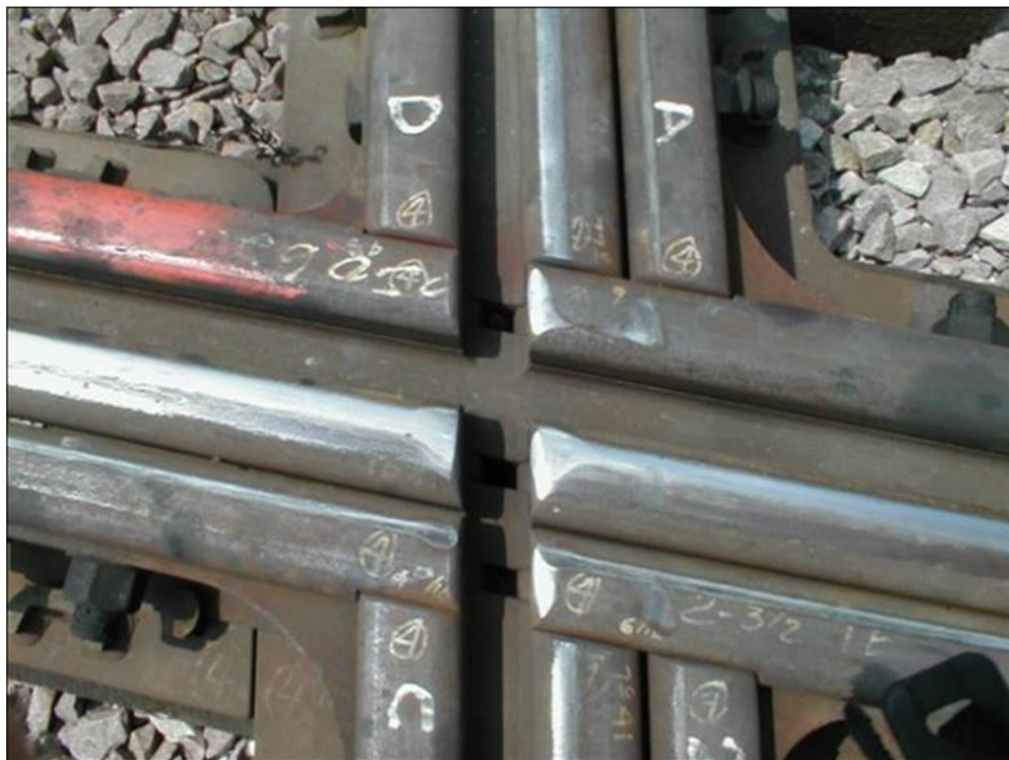
Figure 3. Three-Rail Crossing Diamond
