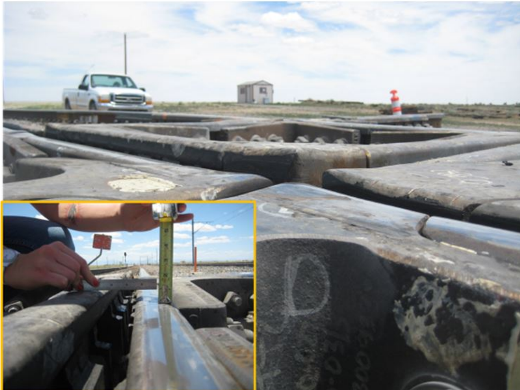
Figure 97. Differential elevation between the guardrail (left) and the running rail (right), about 1 in
