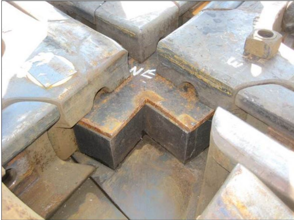
Figure 23. The solid rubber flangeway spacer tile embedded in the Getzner Type B full-coverage rail seat pad resting directly on the platework. The strike plate between the rubber tile and the bottom of the casting corners was designed to protect the rubber.
