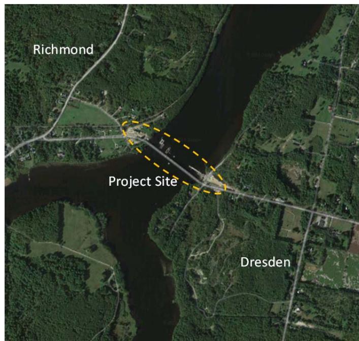
Figure 6.1: Aerial image of the Richmond Dresden Bridge site Route 197 Bridge site showing recent construction of the new bridge on the north side of the existing bridge structure (Google Earth, 2014)
