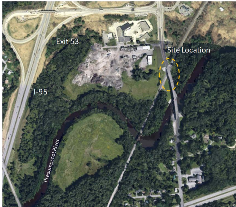
Figure 4.1: Aerial image of the Route 26/100 Falmouth Bridge Site (Google Earth, 2014a).
