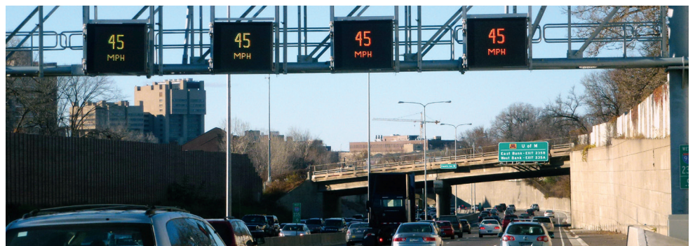
Lessons learned from Minnesota’s use of ATM are informing MDOT’s efforts to install a similar system on US-23. That project, which is expected to be operational in 2018, will improve traffic flow and safety during peak-hour congestion.
