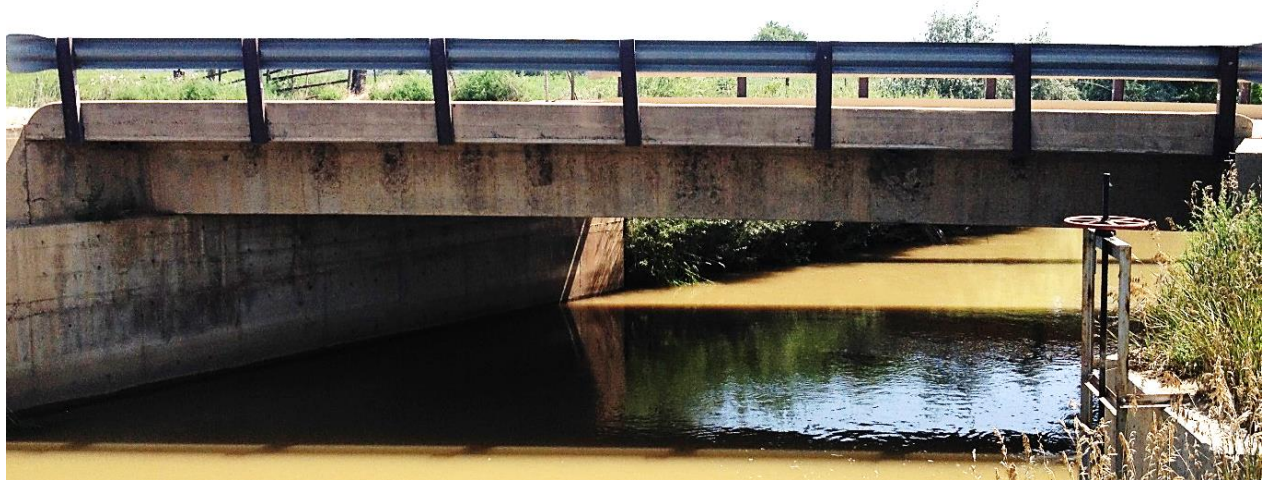
Figure 8.1 Bridge LR3-0.2-50 east elevation view
