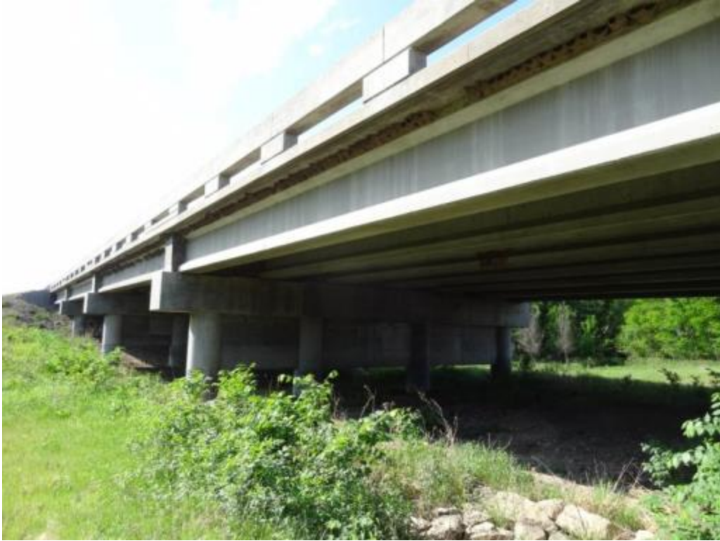
Figure 2.3: Side View of Bridge
