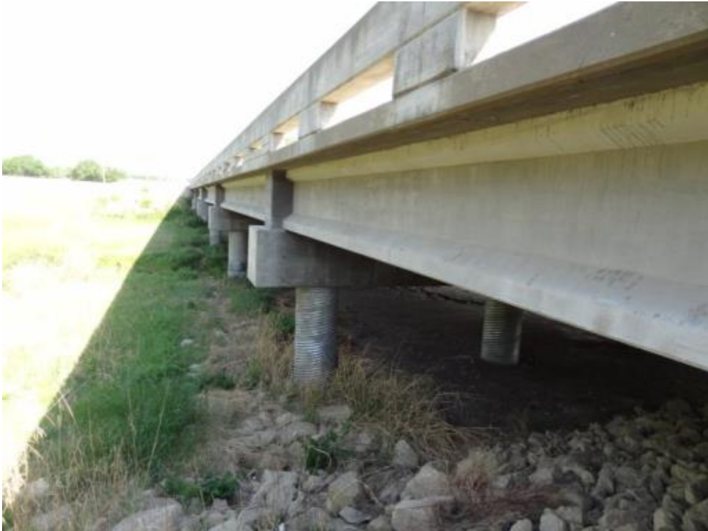
Figure 2.4: Close-Up View of Side of K3 Girders
