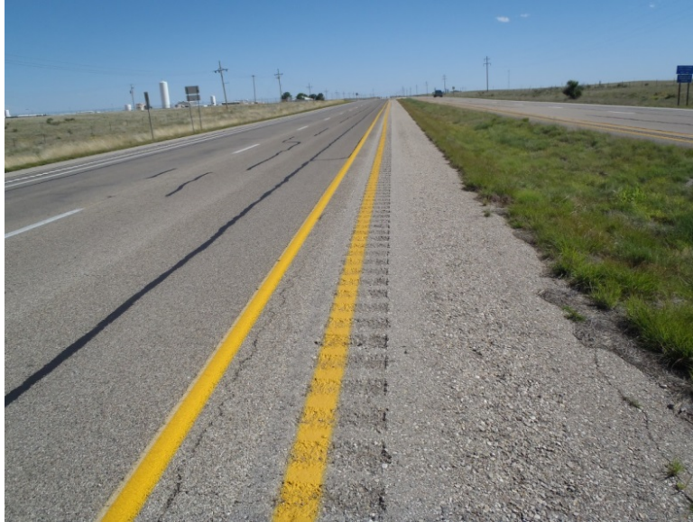
Figure 3-4 Installed Yellow Rumble Stripes (Near Insider Shoulder and Median)
