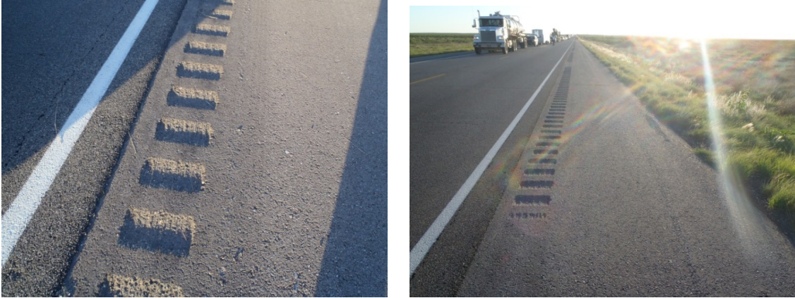
Figure 3-2 Existing Shoulder Rumble Strips on U.S. 285 (within NMDOT D2 Administrative boundary)
