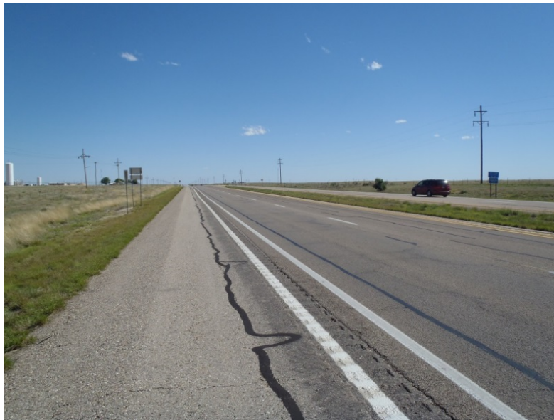
Figure 3-3 Installed White Rumble Stripes (Near Outside Shoulder)
