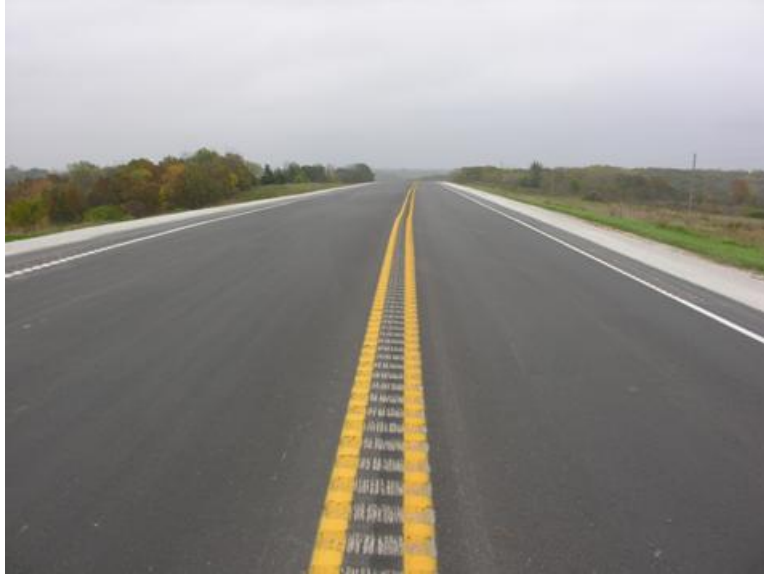
Figure 2-4 Centerline Rumble Strip
