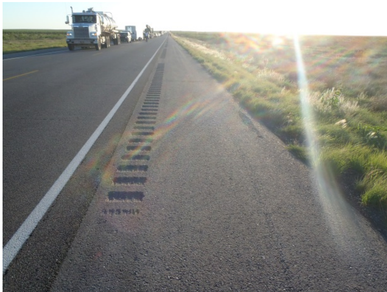
Figure 2-3 Shoulder Rumble Strip
