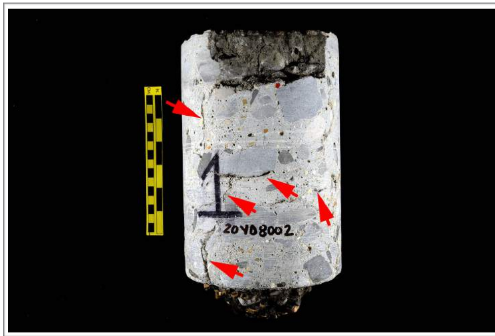
Figure A6. (a) Photograph of the side of the core showing overview of cracks (red arrows). The yellow scale is ~ 150 mm (6 in.) long.
