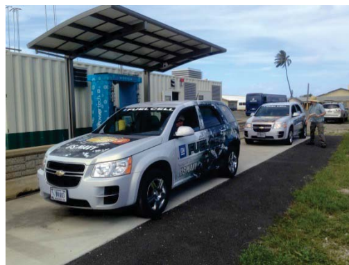
Figure 20. Fast-fill, dual pressure hydrogen fueling station at Marine Corps Base Hawaii (MCBH).
