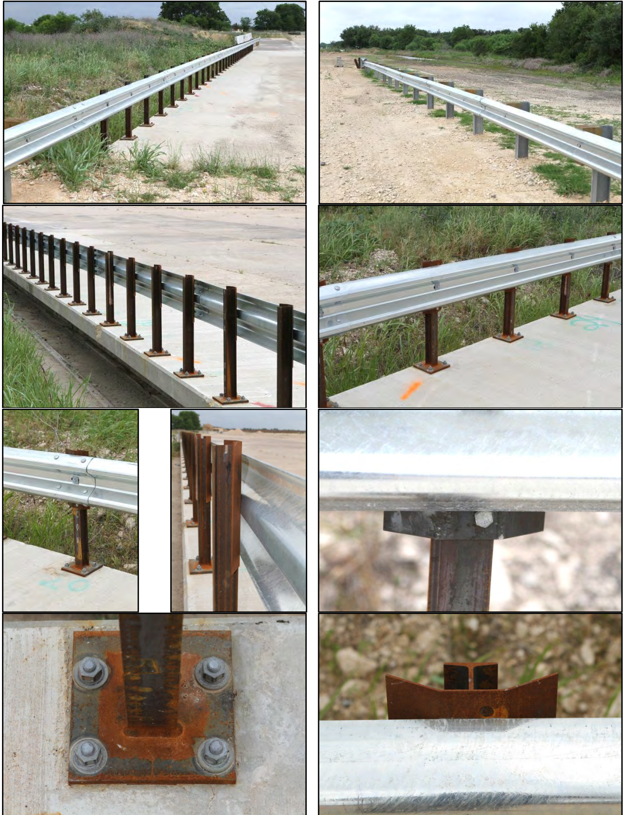
Figure 2.4. TxDOT T631 Bridge Rail before Test No. 490024-1-5.
