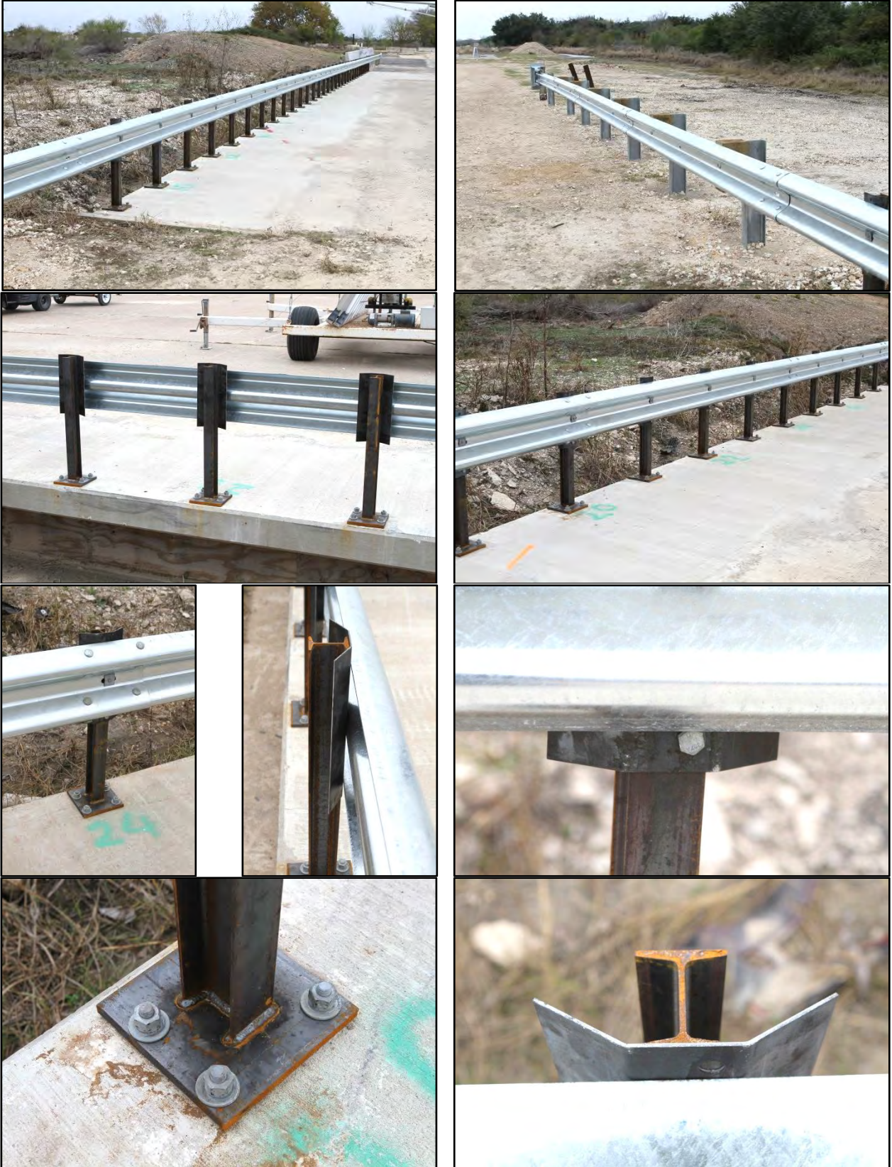
Figure 2.2. TxDOT T631 Bridge Rail before Test No. 490024-1-2.
