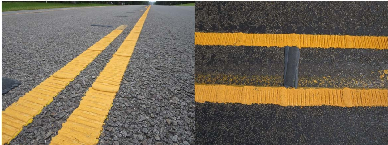
Figure 13. 4-In. Inverted Profile with Audible with Center Line Rumble Bars.
