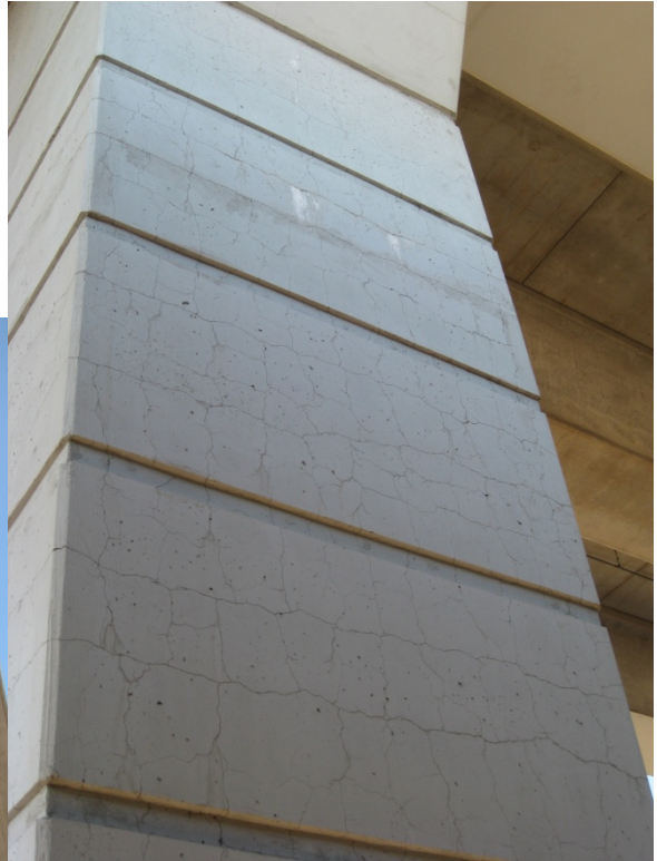
(a) Elevation View and Typical Cracking on Tension Face (Houston, TX).
