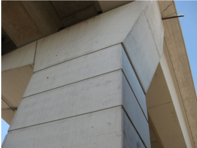
(a) Elevation View and Typical Cracking on Tension Face (Houston, TX).
