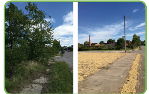
Before and after: Clearing overgrown vegetation revealed a buried sidewalk.
