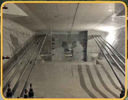
Reinforcements: Steel cables inside the box bridge add strength.
