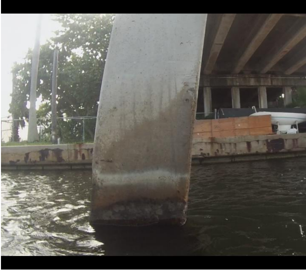
Figure 72: Above water and underwater images of the east-most piling imaged along the southern row of pilings. The conditions of the piling above water and the streambed underwater are visible in the images. At the waterline discoloration and repair work are visible. A long horizontal crack, about a foot above the waterline is visible in the above water image, as are small chipped sections of the corners.
