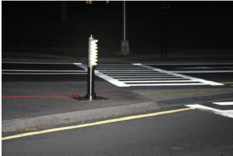
Figure 5. Fluorescent bollard luminaires tested in New York State.
