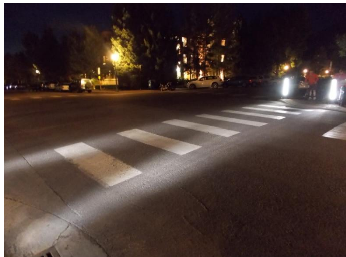
Figure 6. LED bollard luminaires tested in Colorado.
