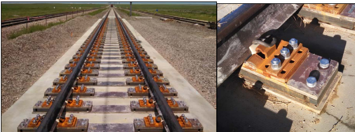
Figure 23. RTT Precision Geometry Slab Track and Adjustable Fastener
