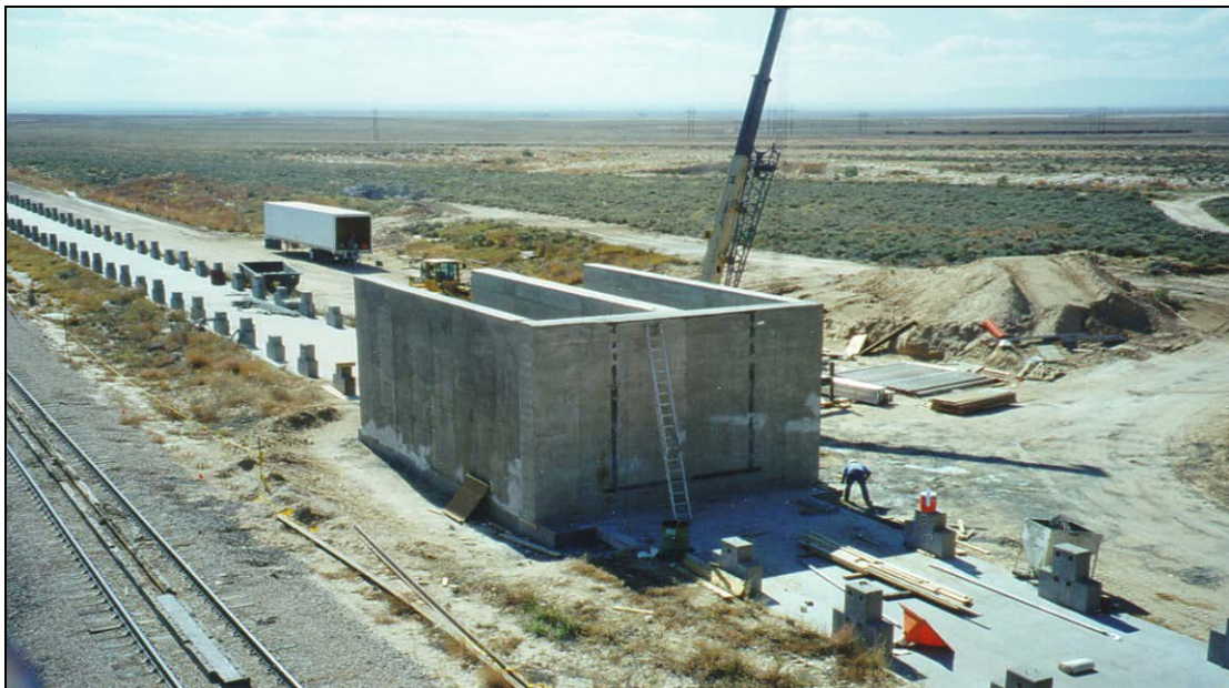
Figure 46. Vehicle Impact Wall Under Construction
