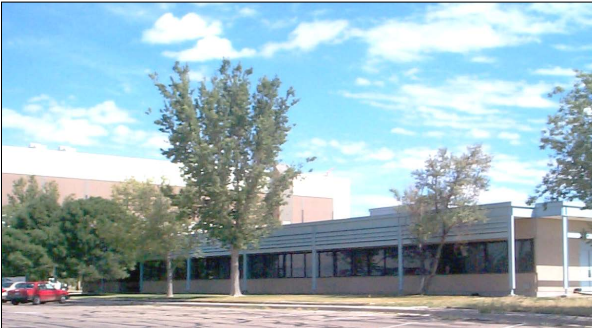
Figure 6. The Project Management Building (PMB)
