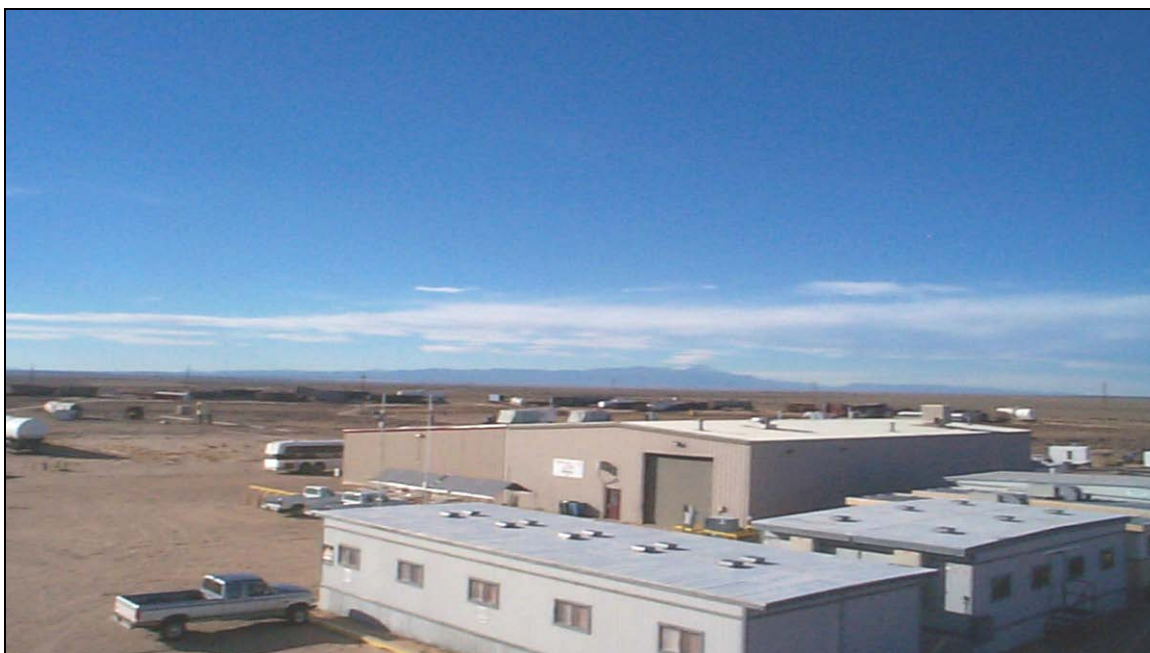
Figure 12. Security and Emergency Response Training Center (SERTC)
