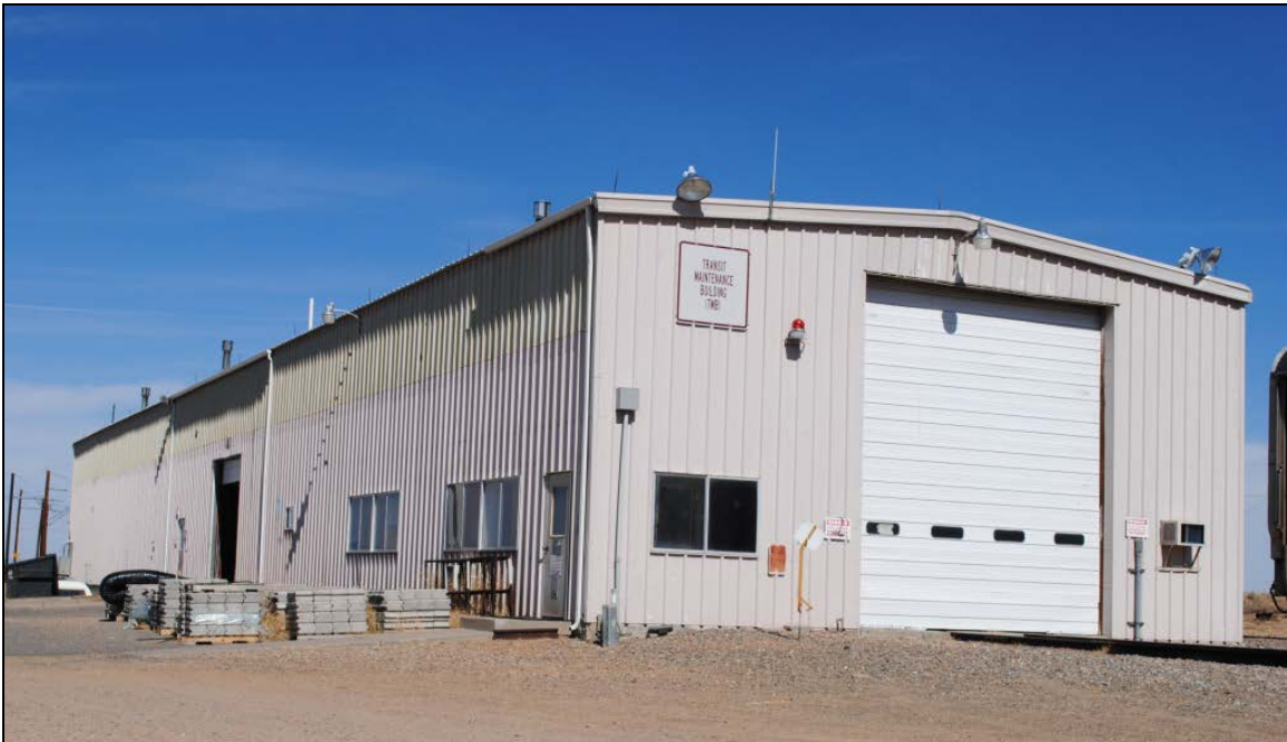
Figure 13. The Transit Maintenance Building (TMB)
