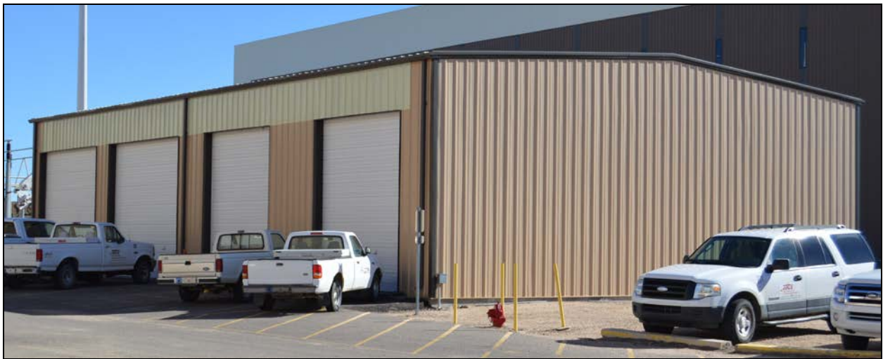
Figure 10. The CSB Storage Building (aka the TTX building)
