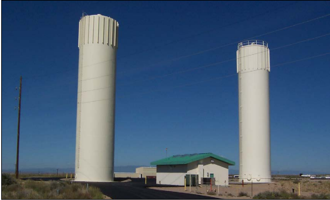
Figure 50. Water Reservoir and Distribution Pump House.
