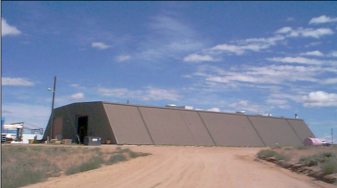
Figure 15. The Urban Rail Building (URB)
