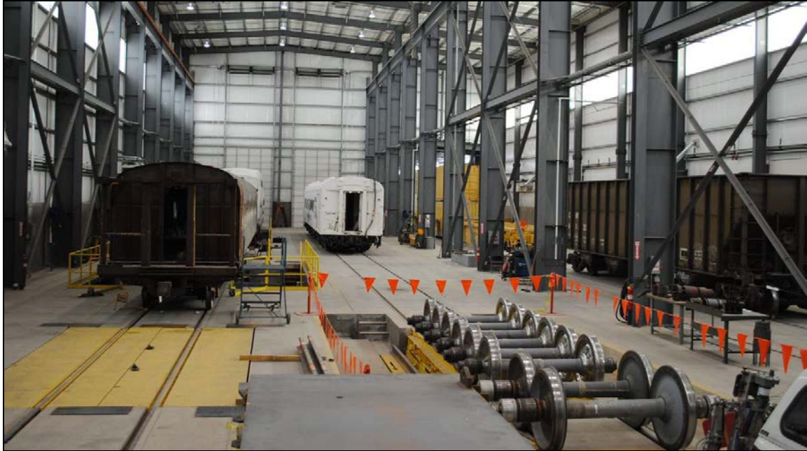
Figure 17. PSB High Bay, Facing South
