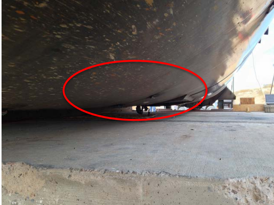
a) Localized jacket/tank transition
