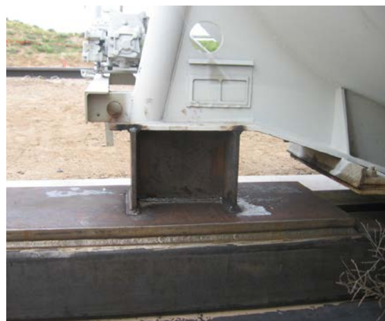
(b) Welded I-beam connection
