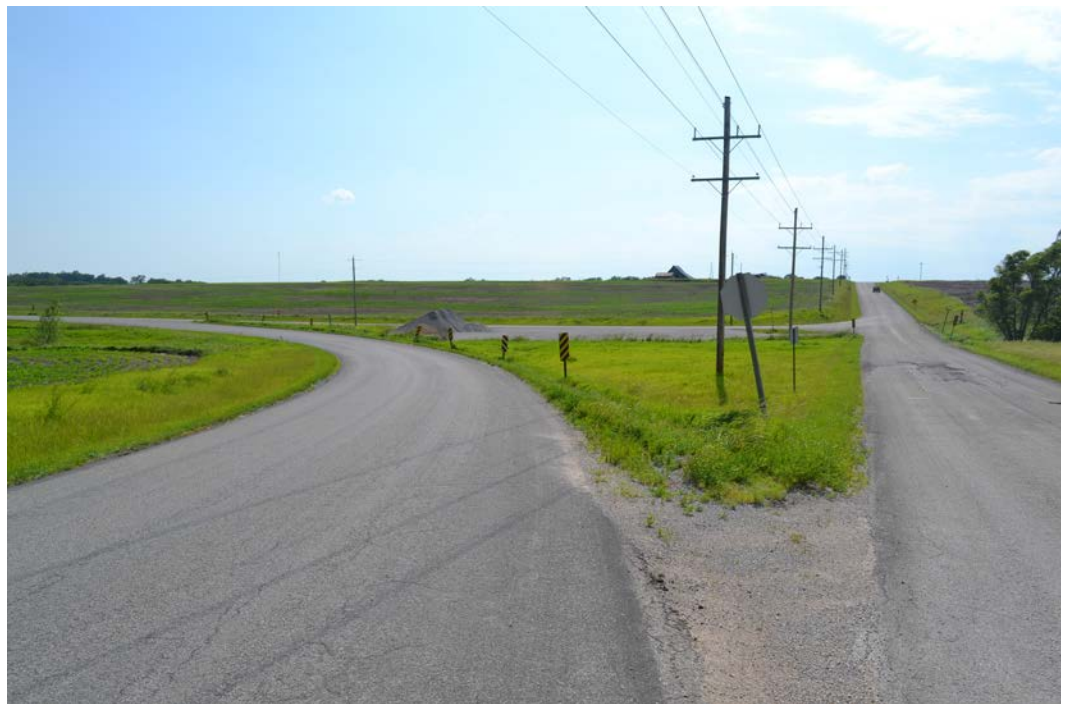
Study Corridor Containing a Horizontal Curve
