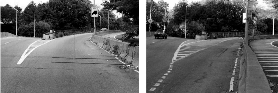
Figure 3 Longitudinal Markings at Experimental Ramp in New York – Before (Left) and After (Right) (11)
