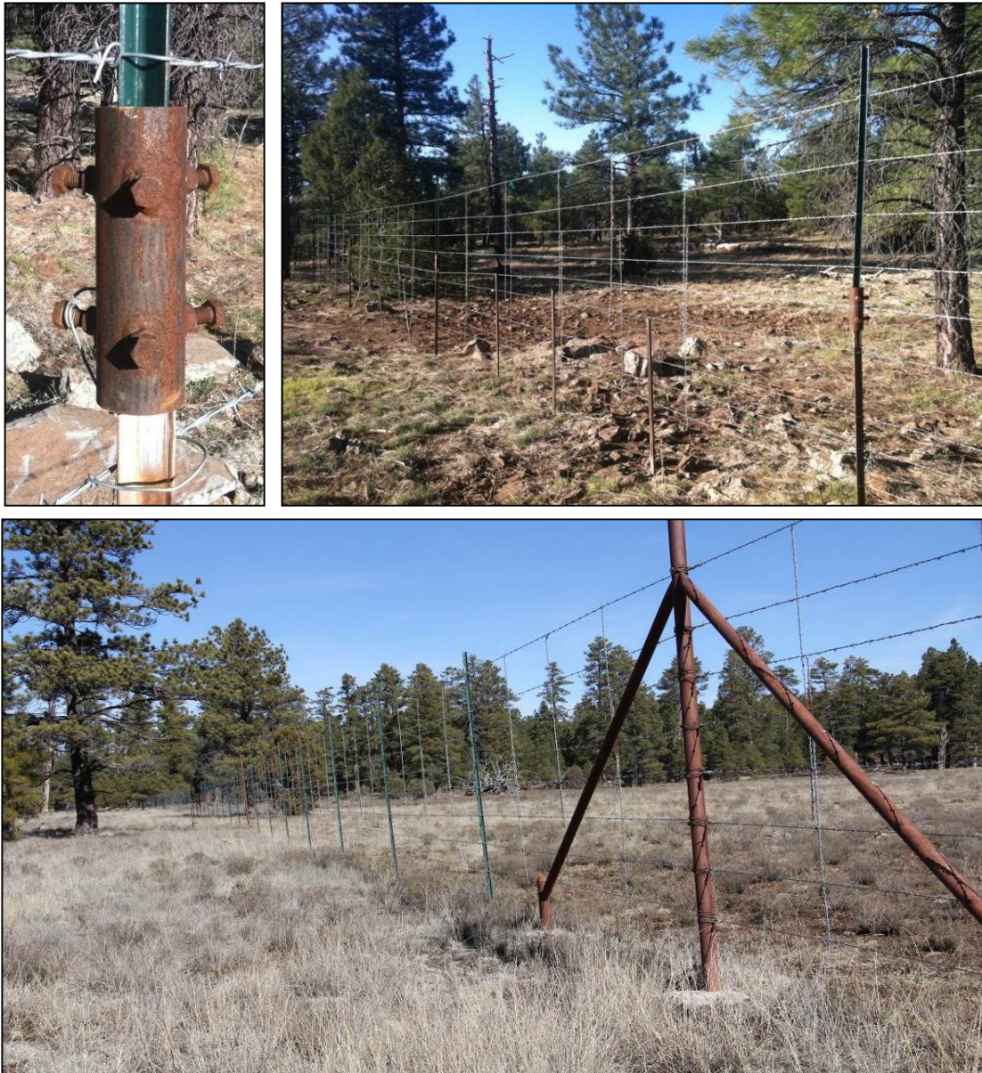
Figure 8. Heightened Fencing along the Study Area: Metal Couplers Attached Extensions to Existing T-Posts (Top Panel); New 8-Ft-High Fencing Replaced Fencing that Was Too Degraded to Heighten (Bottom Panel)
