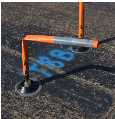
Figure A-15. Sample 8T Failure at 6 Impacts.
