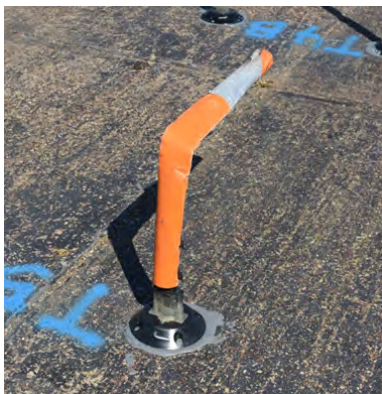
Figure A-9. Sample 5T Failure at 32 Impacts.
