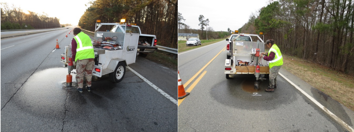
Figure 6—Cutting Cores from Pavement in Cracked and Un-Cracked Areas
