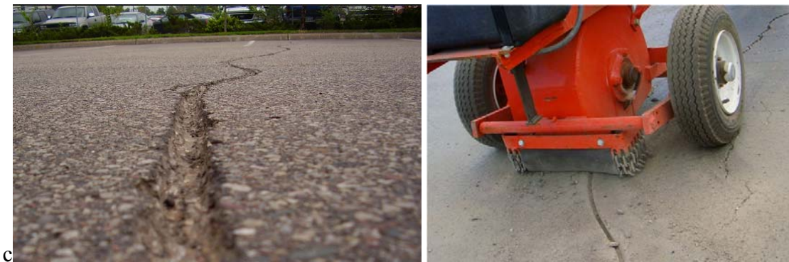
Figure 2.2: Crack after cutting
