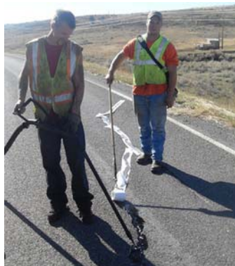
Figure 2.7: Toilet paper as blotting material( http://www.whartonasphalt.com/crack.asp )
