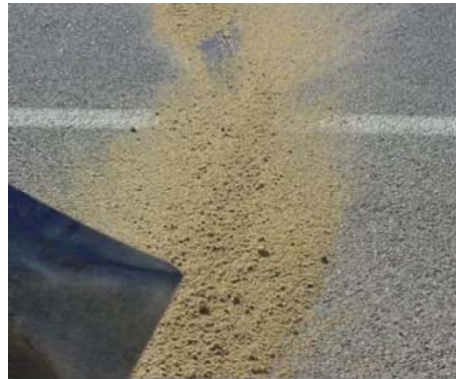
Figure 2.6: Sand as blotting material
