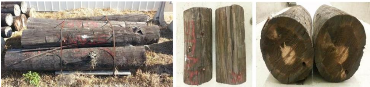
Figure 5-1. Typical red oak pile specimens used in the study.
