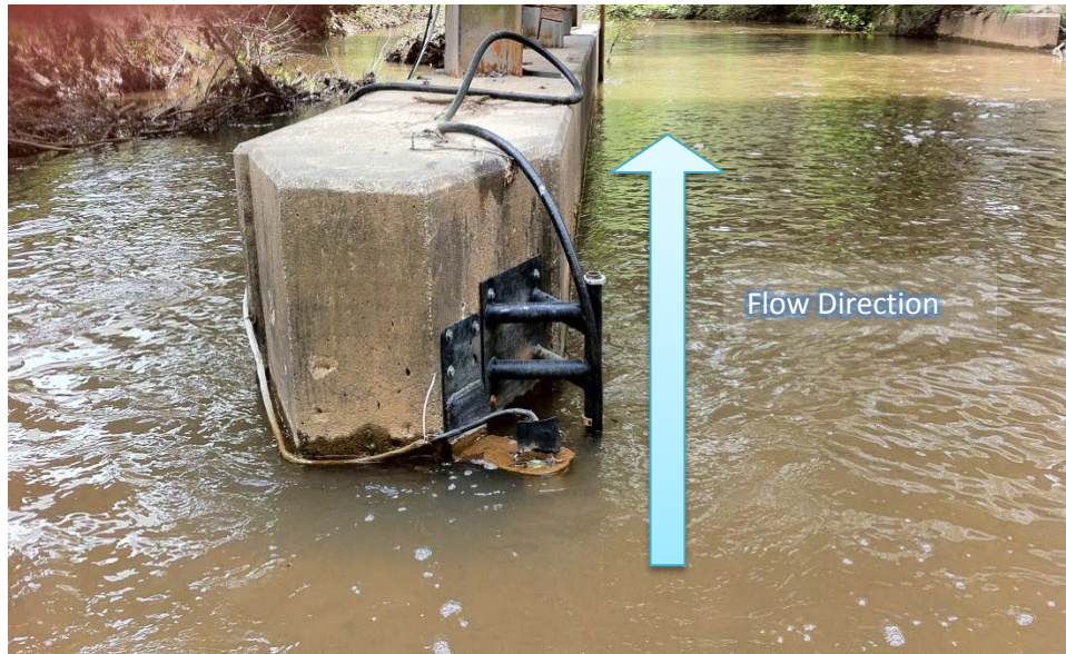
Figure 6.4: Instruments mounted on the face of the footing pad at the pier.
