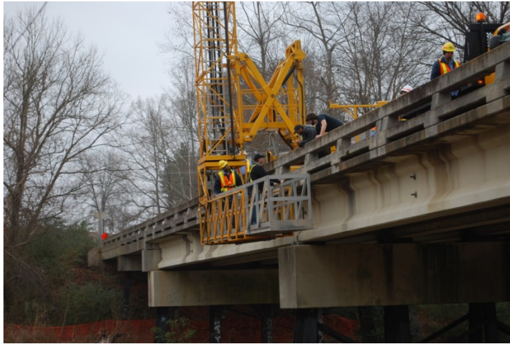
Figure 6.7: SCDOT crew assisting in running the cable at Field Site 2.
