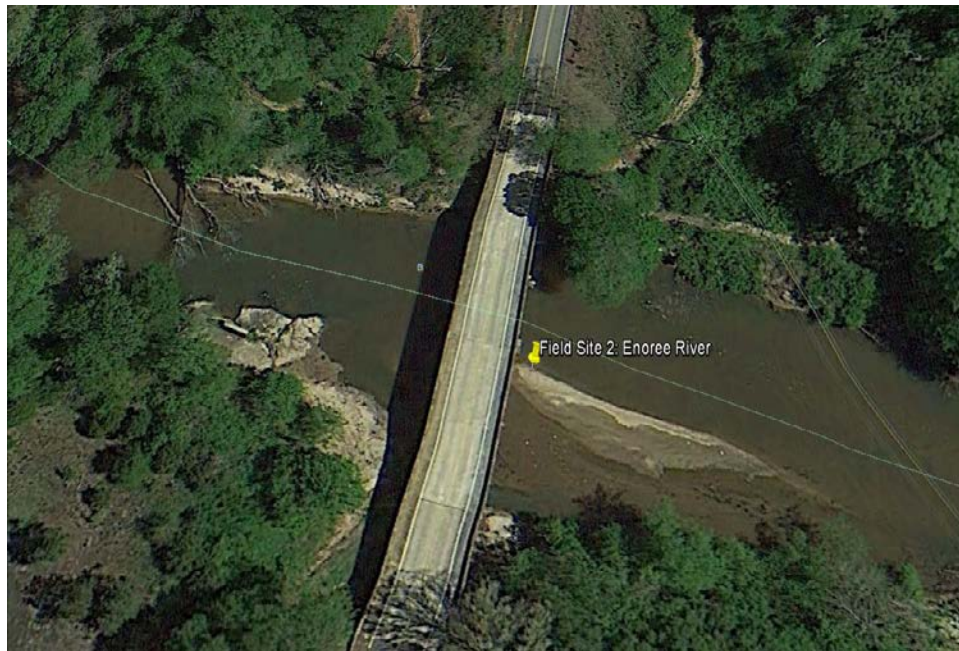
Figure 6.6: TDR and sonar at Field Site 2 (Source: Google Earth).
