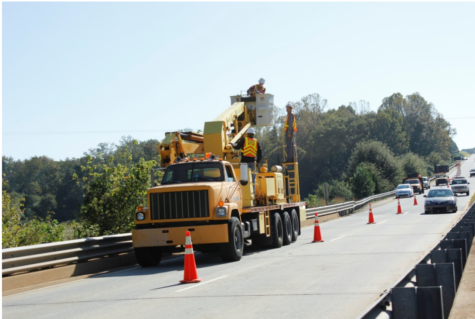
Figure 6.3: SCDOT crew assisting in running the cable at Field Site 1.
