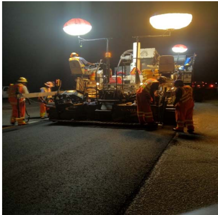
Figure 7-4 Field Test Sections (Night Paving: Hwy 76, Marion County, SC)
