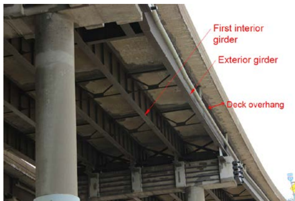
Figure 1.1 Deck overhang in bridge.
