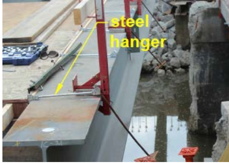
Step 1: Attaching hanger to the girder
