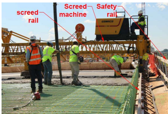
Figure 2.4 Screed rail placed on the overhang formwork.
