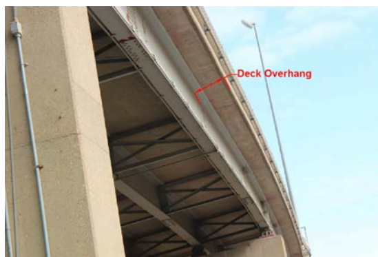
Figure 2.1 Deck overhang in a steel girder bridge.
