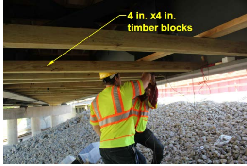
Figure 2.7 Timber blocking in addition to transverse tie bars.
