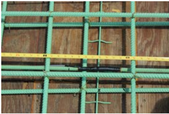
(a) Strain gage in the transverse tie bar
