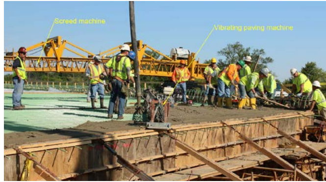
Figure 3.19. Vibrating paving machine and the screed machine during construction.
