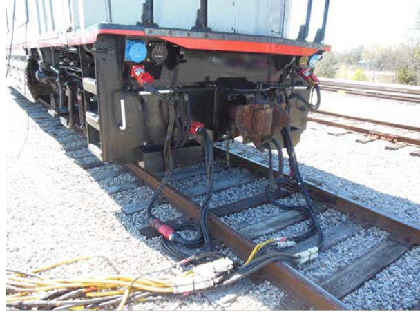
(b) Load Box Cables Connected to the Locomotive
