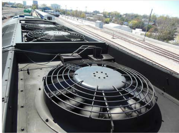
(d) Exhaust Sampling Lines Inserted Into the Head End Power Engine Exhaust Duct
