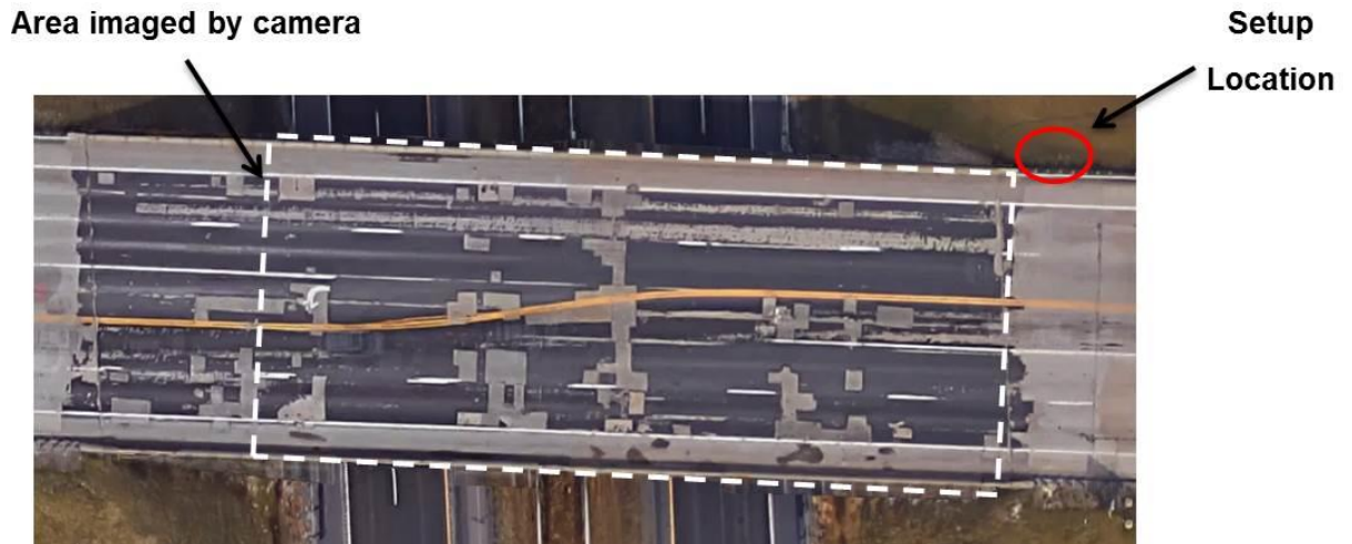
Figure 32. Aerial view of the Grindstone Bridge.
