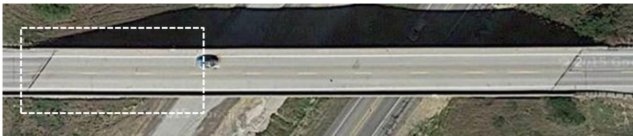
Figure 18. Aerial view of the Iowa Bridge deck showing area imaged by the IR-UTD.
