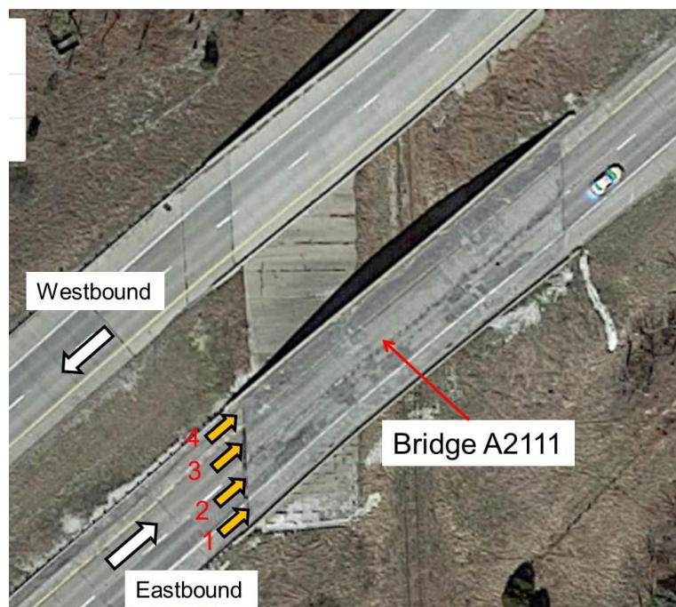
Figure 53. Aerial view of Bridge A2111 in Fulton, MO.
