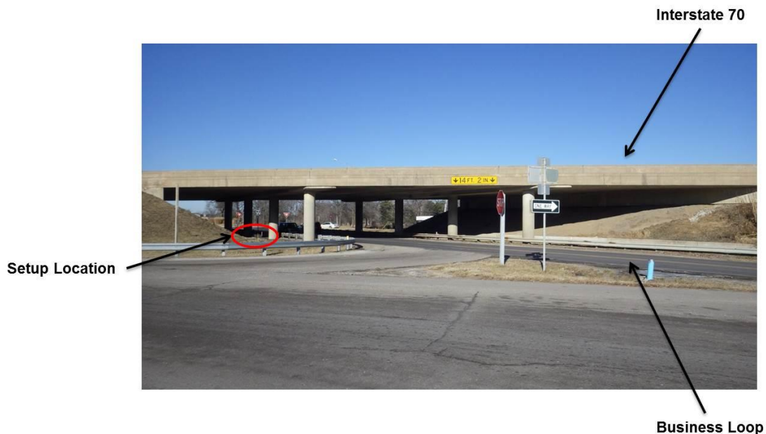
Figure 45. Photograph of the West Blvd Bridge illustrating the test set-up location.
