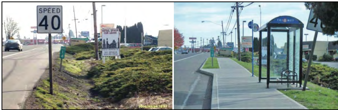
Figure 31. SW Oak & 17th – Before (Left) and After (Right) for Line 57-TV Highway Improvement
