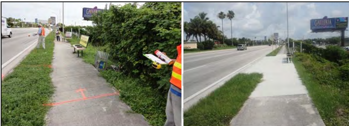
Figure 5. (Left) Bus Stop Before Reconstruction for ADA Accessibility (Right) Bus Stop Following Reconstruction
