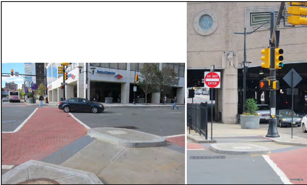
Figure 28. Grade Cut-Through Provides a Design Solution Where Three Pathways Meet. Newark Penn Station, Newark, NJ
