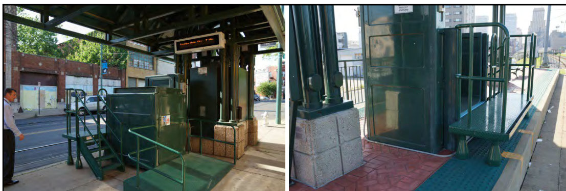
Figure 22. (Left) Trolley Station with Mechanical Lift and Variable Message Sign; (Right) Trolley Station Wheelchair Boarding Platform and Textured Ground Surface
