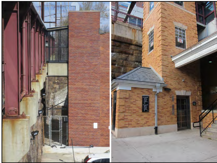
Figure 26. (Left) Old Inbound Elevator; (Right) New Inbound Elevator, New Brunswick Station, New Brunswick, NJ
