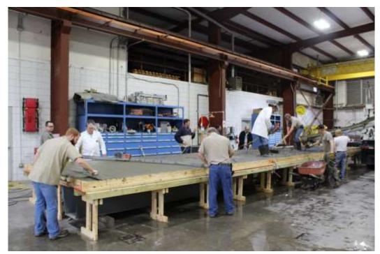
Figure 3-9 Casting the concrete deck.
