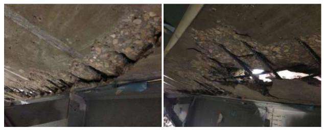
Figure 4-20 Punching in the bottom of the deck.
