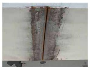
Figure 1-3 Bottom flange cut after the explosion (Source: FHWA Report No FHWA/TX-10/9-5498-1).
