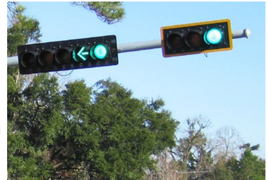
A proven safety countermeasure is the retroreflective border (right) that helps a signal stand out from its background, especially at night, dusk, and dawn.
