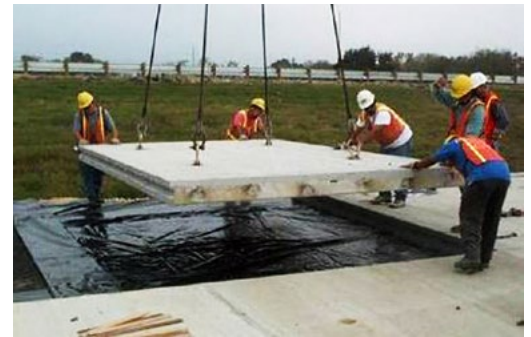
Workers lower a temporary, precast concrete slab into place.
