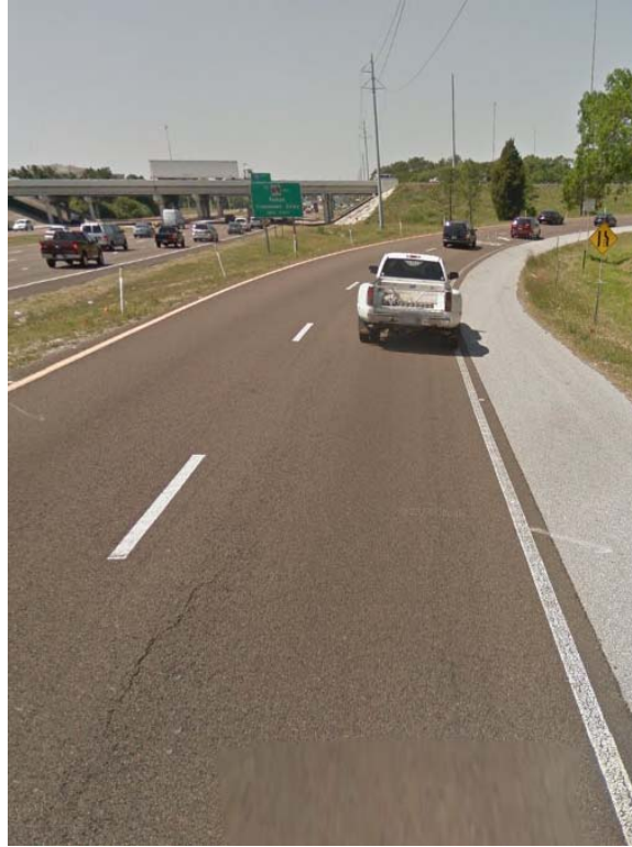
Figure C.5 – Completed HFST (May 2011).
