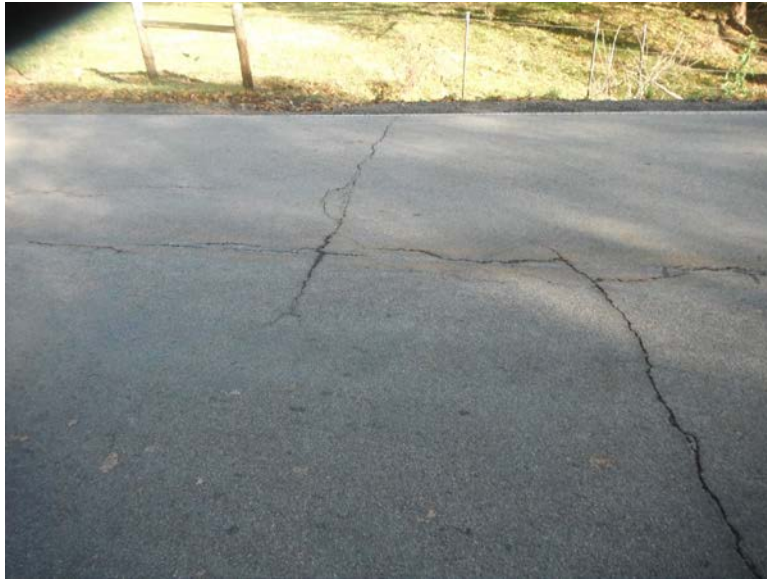
Figure 2.17 – Reflective cracking
