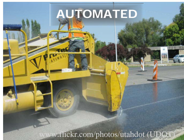
Figure 2.5 – Aggregate spreading
