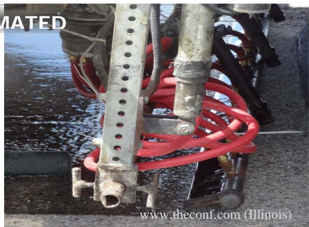
Figure 2.4 – Binder spreading
