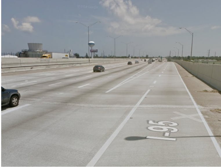
Figure C.15 – Existing surface. (www.google.com/maps/)
