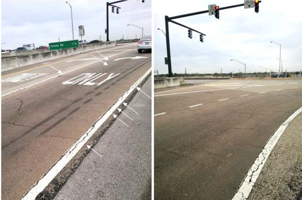
Figure 2.13 – Substrate tearing at an approach (transverse) and around curve (random) (Boca Raton-I-95 to Congress)
