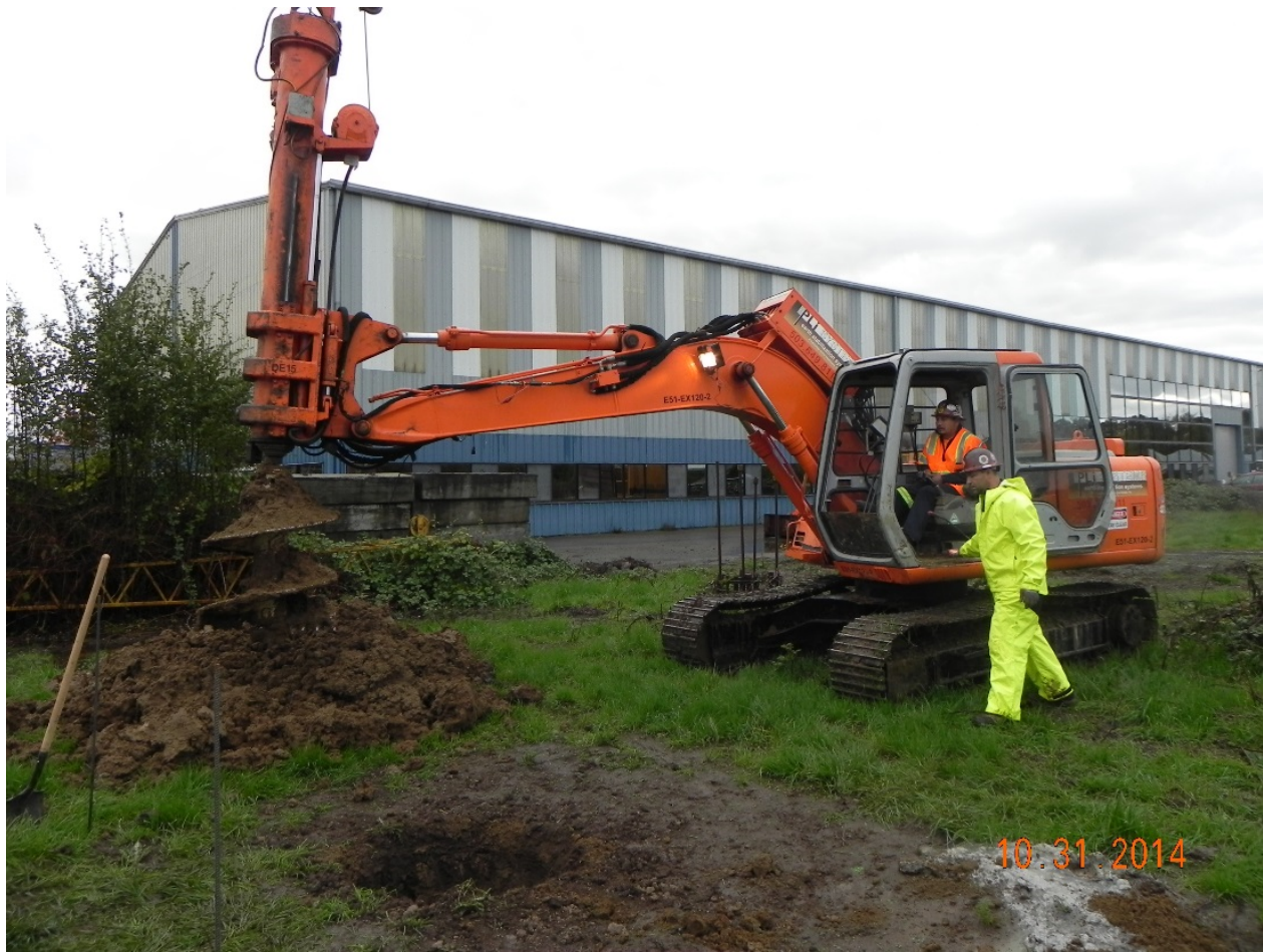
Figure 4.9: Excavating hole using excavator mounted drilling machines
