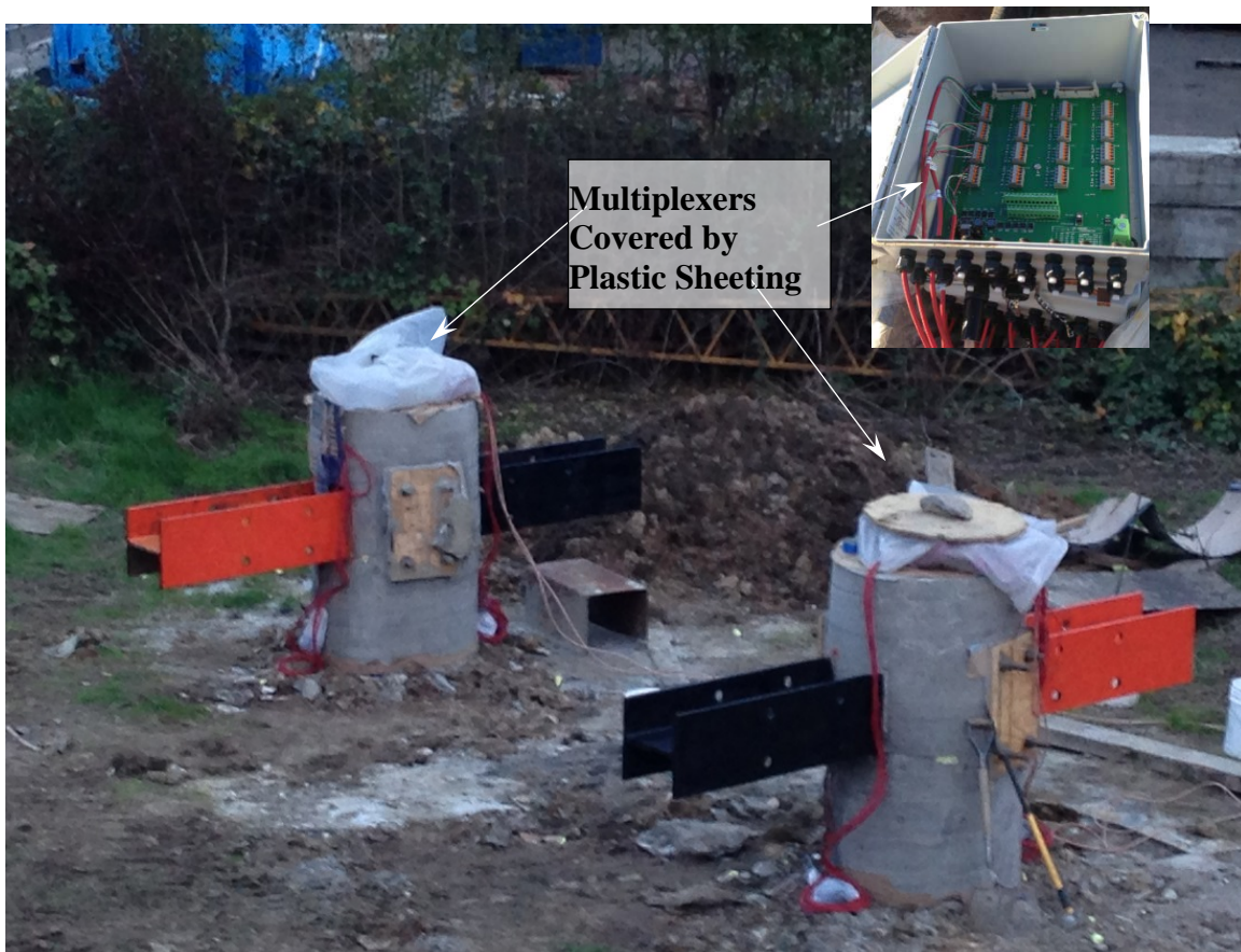
Figure 4.14: Test shafts after construction
