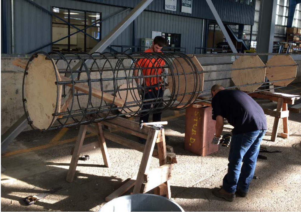
Figure 4.3: Fabrication of a steel cage used in the test shafts
