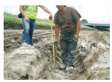
Weak subgrade soils may lead to significant failures under construction traffic loading.
