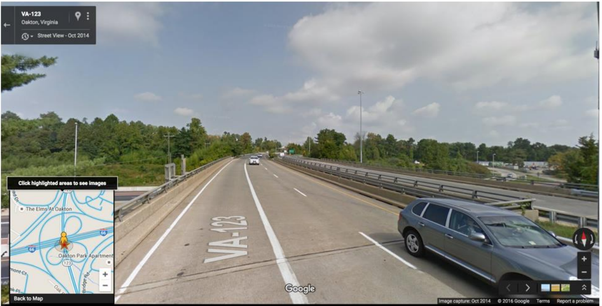
Figure 27. South (top) and north (bottom) views from RSE ID 8 location.
