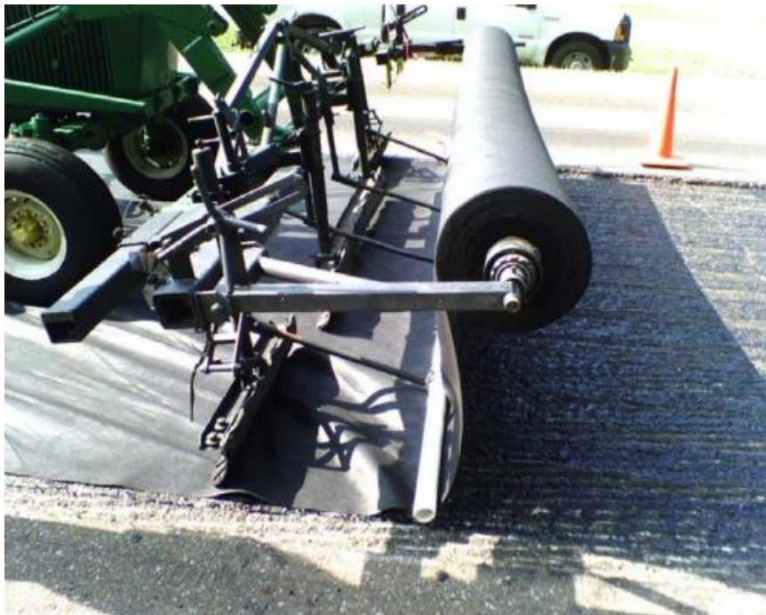
Figure 5.3 Placement of Paving Fabric
