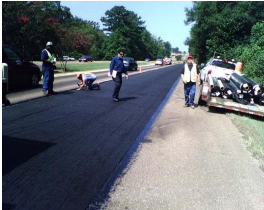
Figure 5.5 Engineer Inspecting of Fabric after Placement
