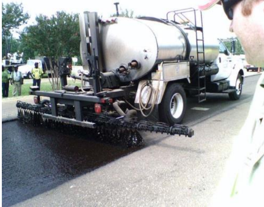
Figure 5.1 Applying Uniform Tack Coat on Test Section
