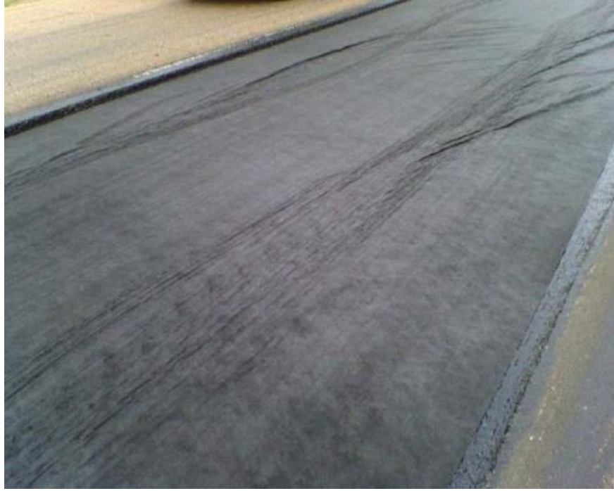
Figure 5.4 Wrinkles after Placement of Fabric
