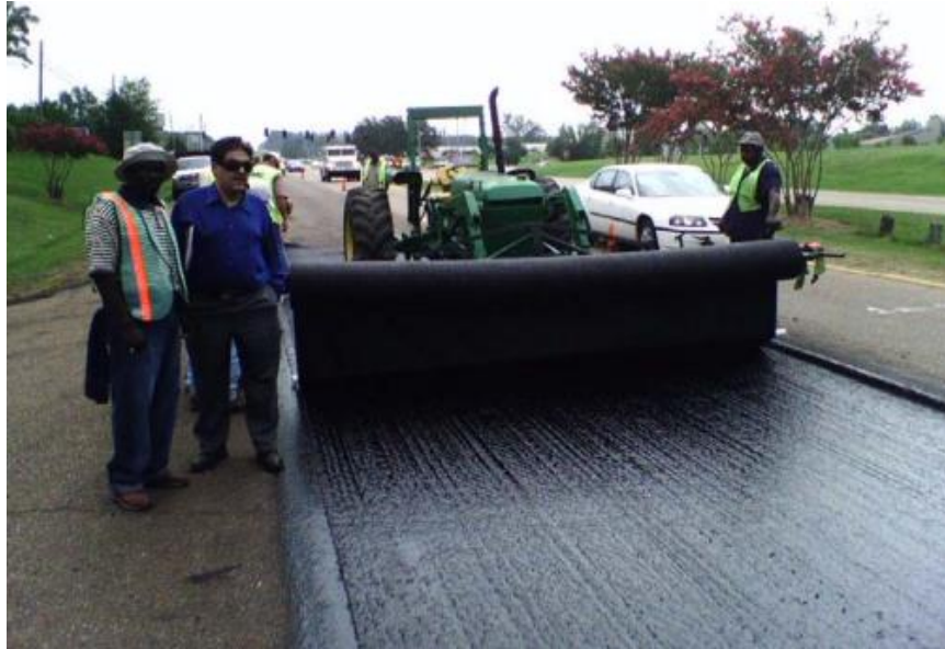
Figure 5.2 Placing Fabric on Test Section
