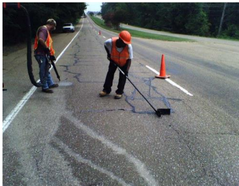
Figure 7.1.4 Sealing Cracks in Section 7
