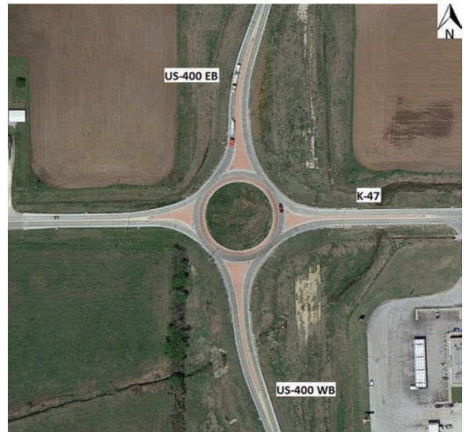
Figure 1.1 US-400 and K-47 roundabout near Fredonia, KS (Google Earth).
