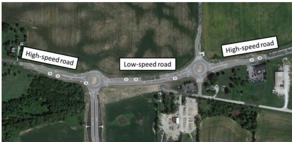
Figure 4.3 SR 32-38 roundabouts in Noblesville (Google Earth).
