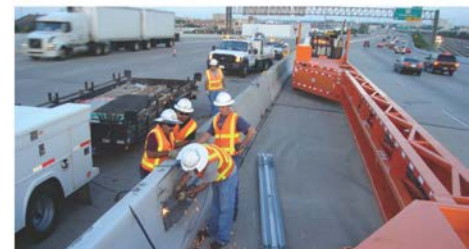
Protected Space Example Mobile Barriers MBT-1
