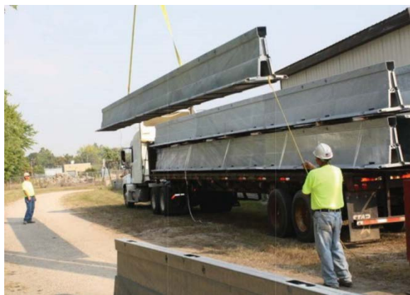
Steel Barrier Installation
