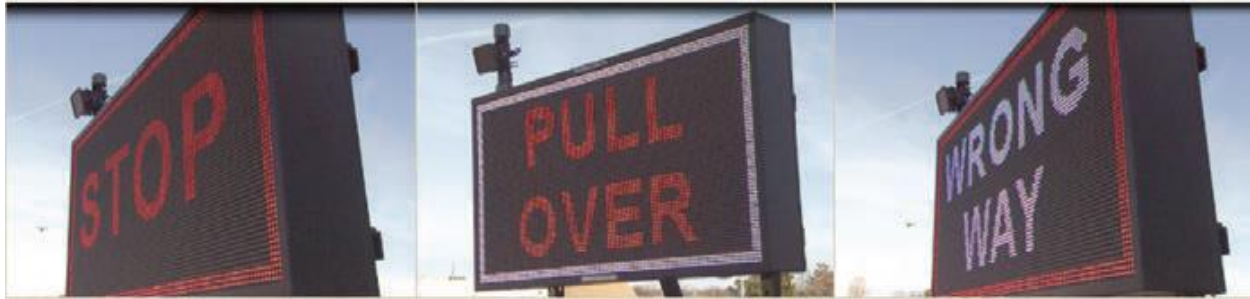
Figure 26. New York Thruway Wrong-Way Entry ITS Warning System (27).
