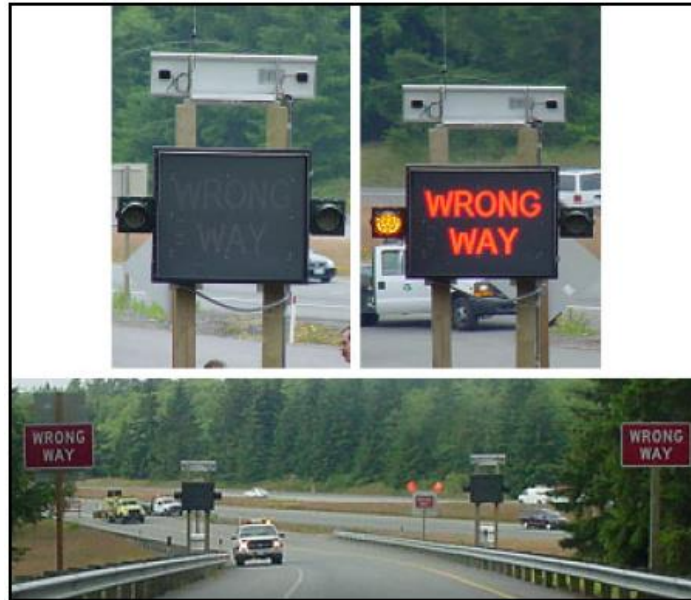
Figure 5. Washington State Wrong-Way ITS System on an Exit Ramp (4).
