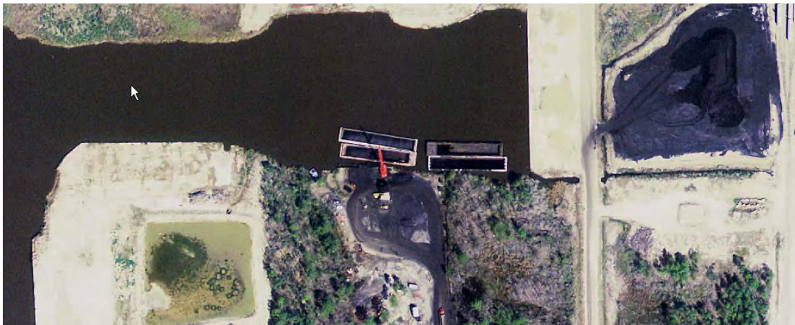
Figure 4 Unloading of Coal at Bienville (courtesy of Google Earth)
