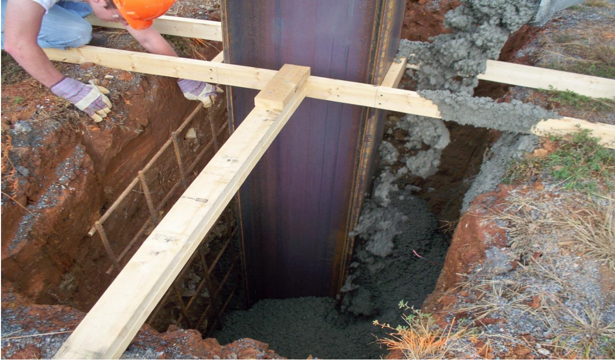
Figure 25. Concrete being poured from a ready mix truck.
