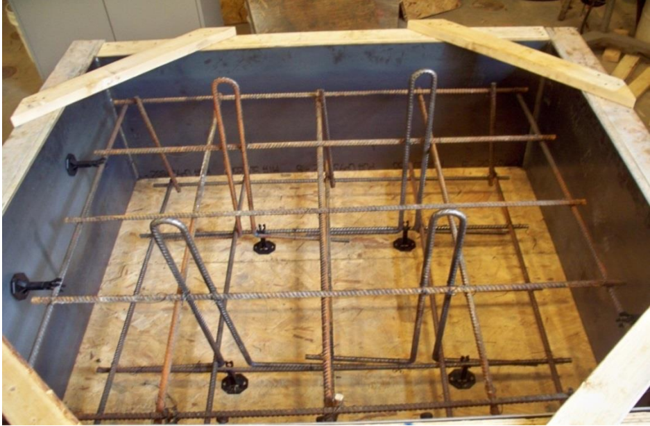
Figure 6. Concrete Block formwork. Showing steel plates, rebar mats and lifting hooks.
