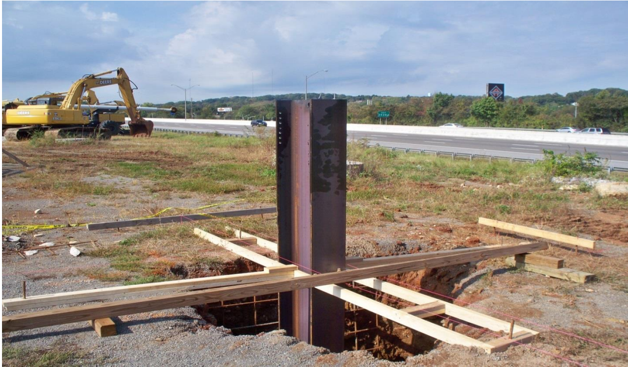
Figure 24. Steel beam sitting within the guide system.
