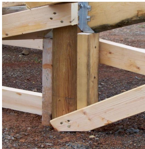
Figure 19. Added 2x4's for extra compression reinforcement.
