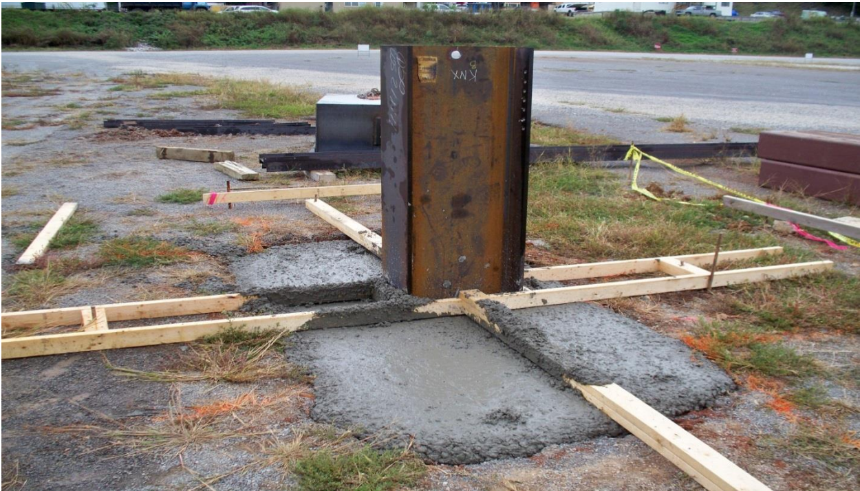
Figure 26. Finished concrete footing.
