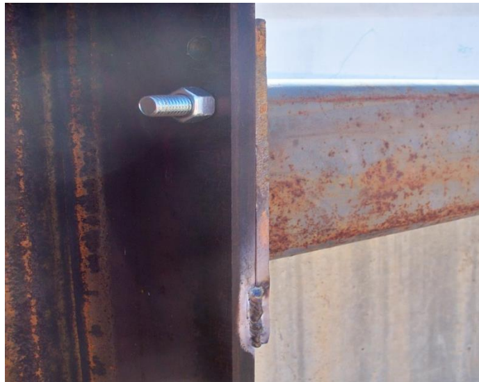
Figure 28. Connection of HSS tubes to vertical beams.
