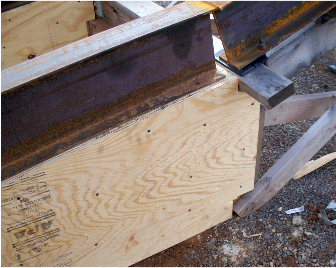
Figure 37. Plywood on the outside of the wall screwed into plywood.
