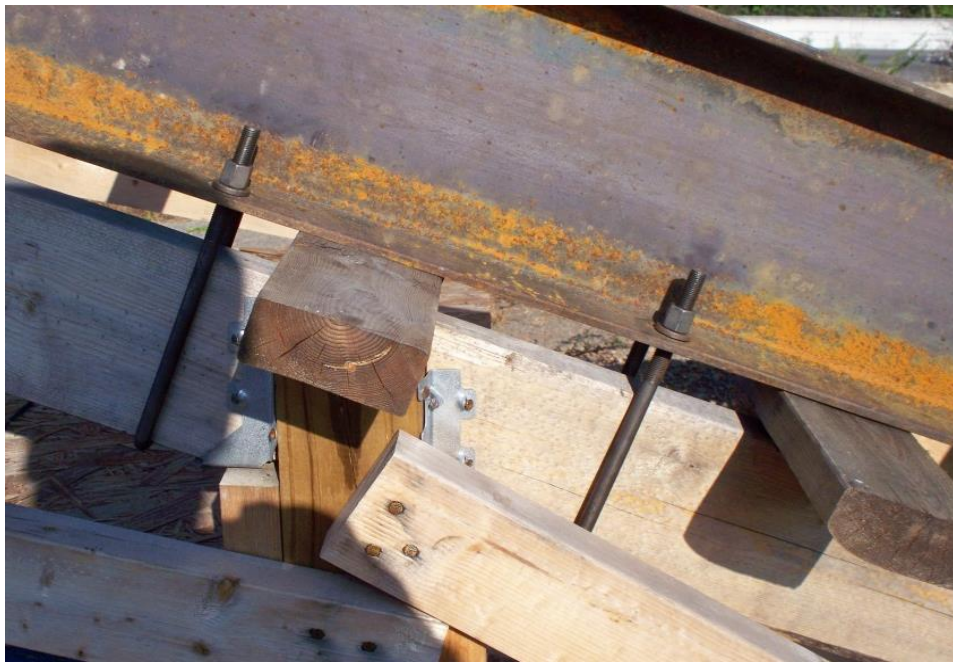
Figure 16. Rails connected to joist by U-Bolts.
