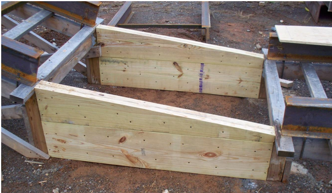
Figure 36. Replacement 2x12 and plywood walls.
