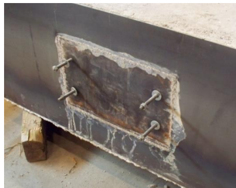
Figure 8. Imbed plate and attachment bolts.
