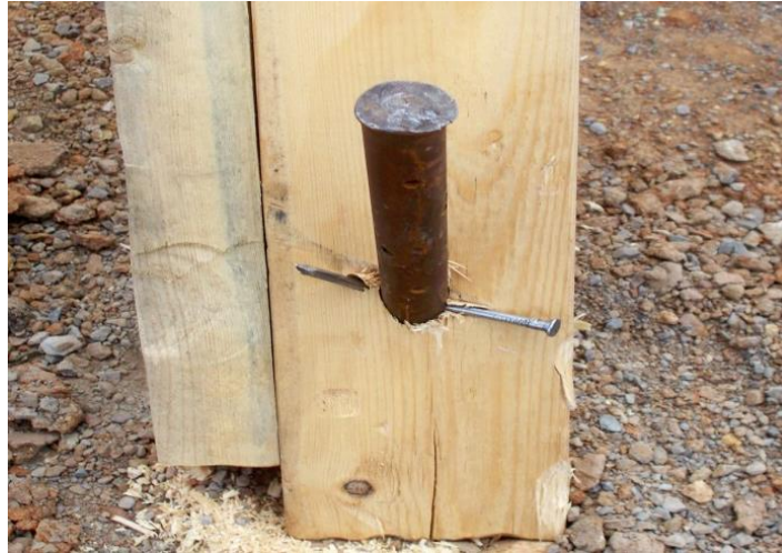
Figure 14. Nail through nail pin. Lateral bracing to ground connection.
