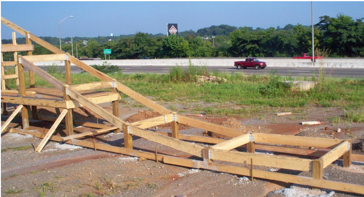
Figure 12. Lower portion of track with top joists prior to 2x4 decking.
