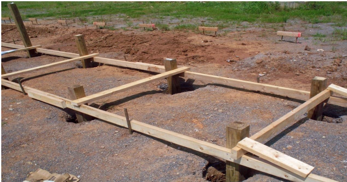
Figure 10. Posts screwed into guide boards.
