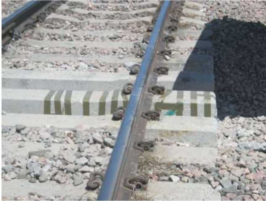
Figure 3.11 Installation of inoperable MBTSS sensors to qualitatively test various protection schemes
