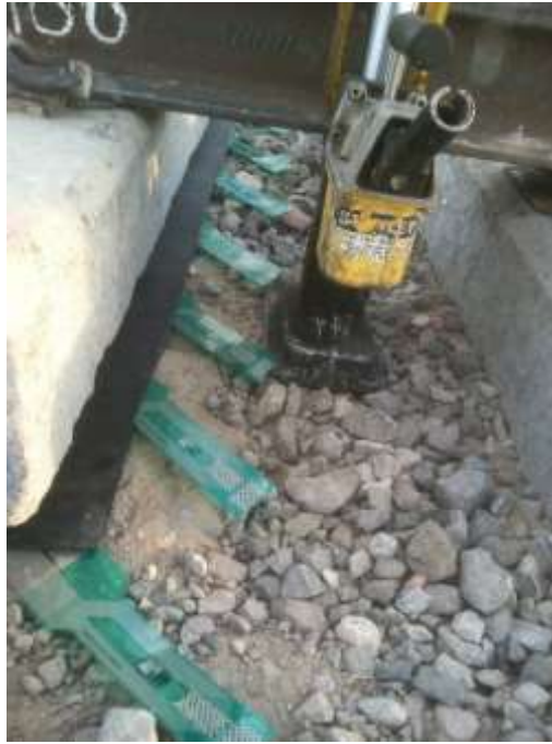
Figure 7.5 Pressure sensors being installed under raised track
