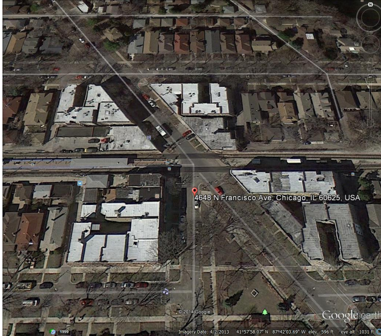
Figure 13 - Manor Avenue crossing (view from above)
