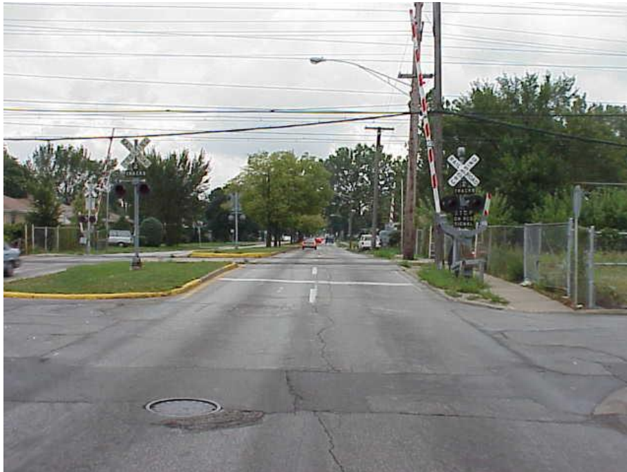
Figure 10 - Crawford Avenue crossing (street view)
