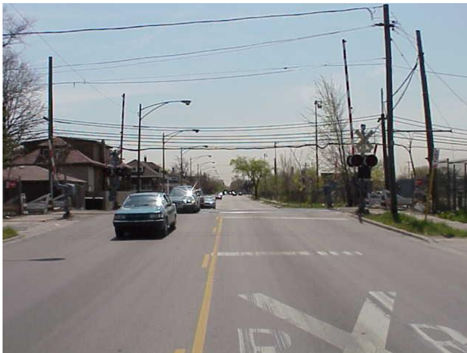
Figure 6 - Kostner Avenue crossing (street view)
