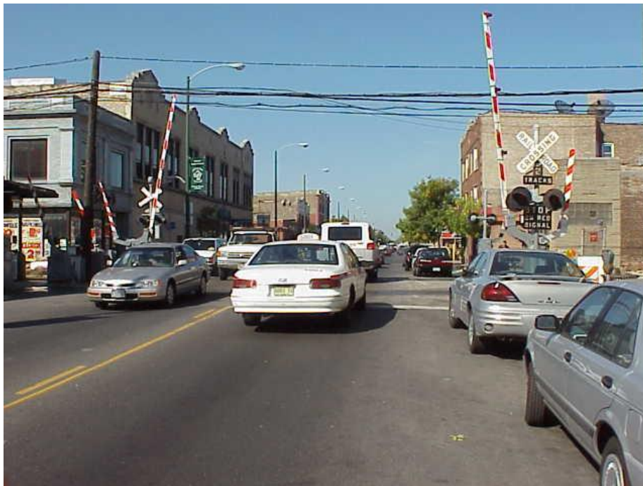
Figure 12 - Kedzie Avenue crossing (street view)
