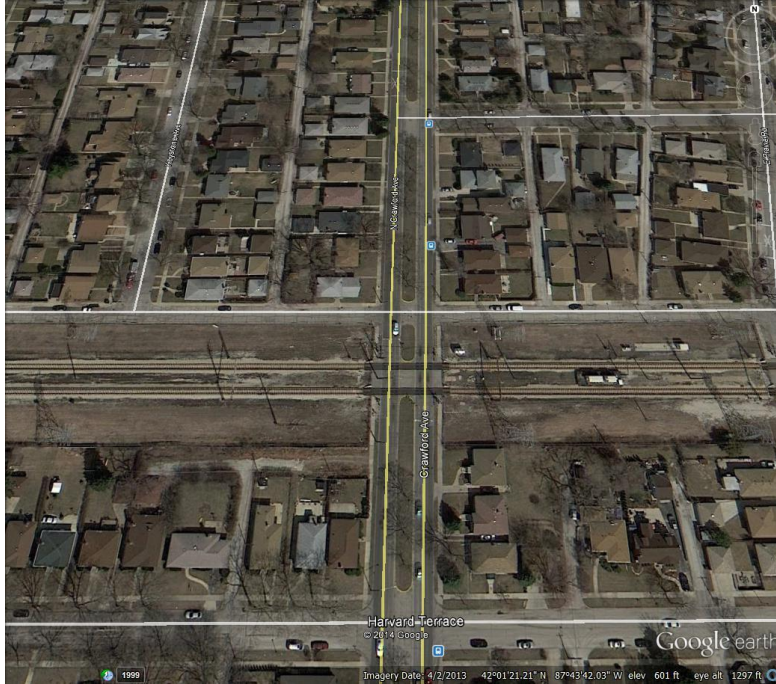
Figure 9 - Crawford Avenue crossing (view from above)
