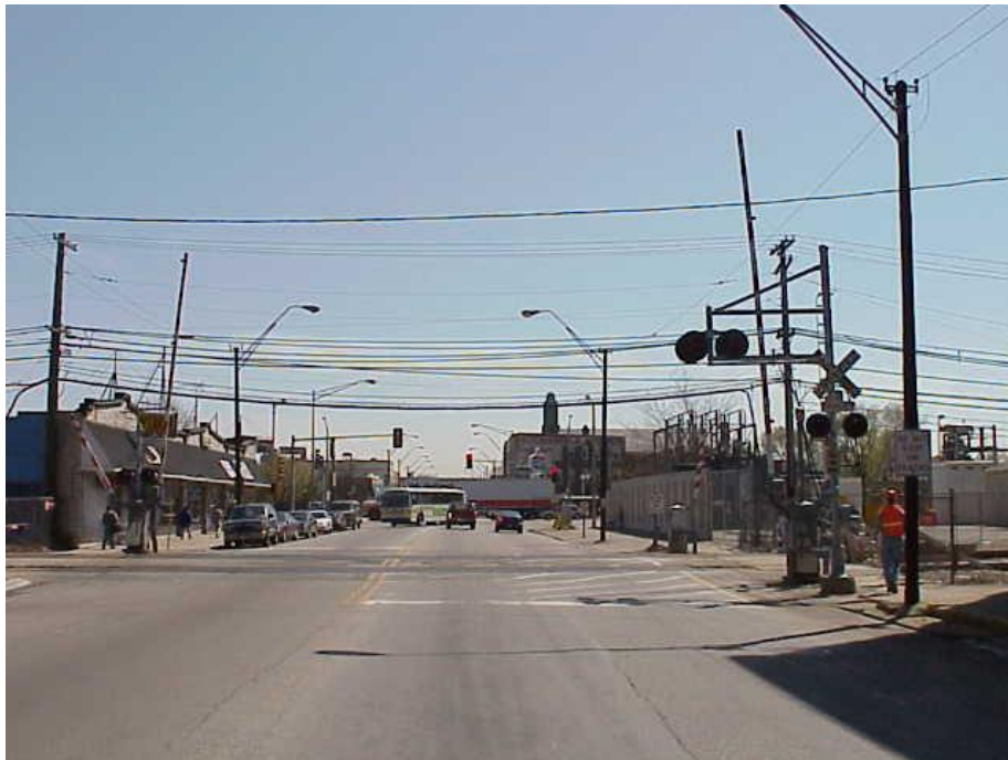
Figure 2 - Laramie Avenue crossing (street view)
