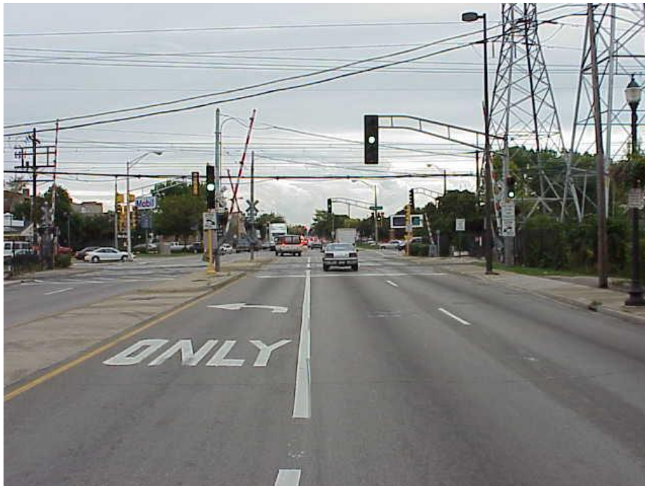
Figure 8 - Oakton Street crossing (street view)
