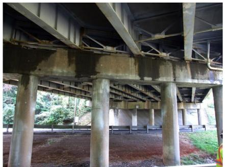
Figure 12. Pier 2 Under 5th Street Extended Bridge Showing Moisture Attributable to Leaking Joint Above Treated Cap and Columns
