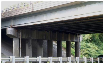
Figure 14. Pier 3 Columns Under 5th Street Extended Bridge: Left 3 columns treated with ECE and sealed; 4 right columns served as control (untreated and not sealed). ECE = electrochemical chloride extraction.
