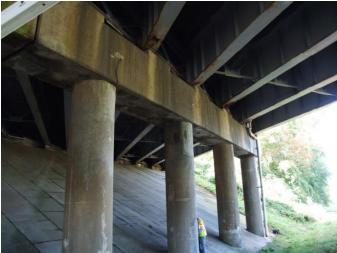
Figure 10. Portion of Pier 1 Under 5th Street Extended Bridge That Was ECE Treated and Silane Sealed. ECE = electrochemical chloride extraction.
