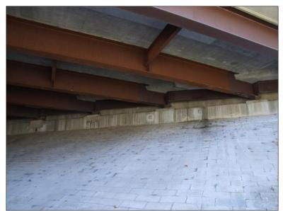
Figure 32. Abutment Under I-95 Bridge Over Hermitage Road After Superstructure Replacement Completed
