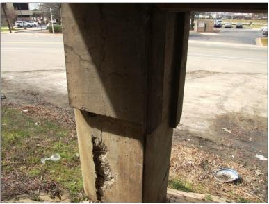
Figure 33. Corrosion Damage Resulting in Spalling of Column Supporting I-95 Bridge Over Hermitage Road Before Repair
