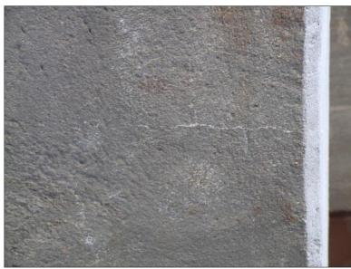
Figure 44. I-95 Bridge Over Overbrook Road Showing Mineral Deposit on Column After ECE. ECE = electrochemical chloride extraction.
