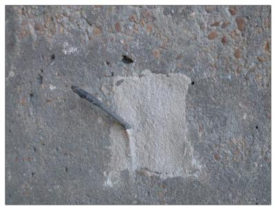
Figure 45. I-95 Bridge Over Overbrook Road Showing Connection Protruding After Completion of ECE Corrosion Mitigation Work. ECE = electrochemical chloride extraction.
