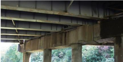
Figure 13. Pier 2 Under 5th Street Extended Bridge That Shows Some Moisture on Untreated Cap Also Exhibiting Some Delaminations That Have Been Repaired
