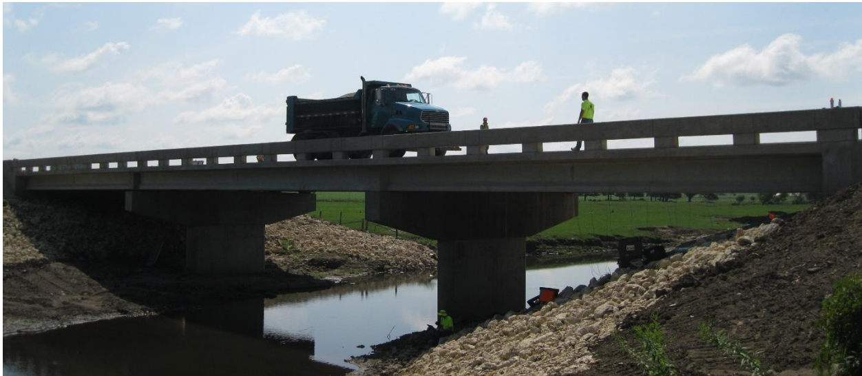
Figure 12. Live load testing of LWFA bridge, 2013
