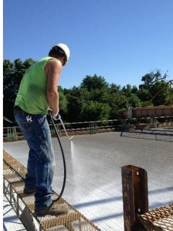
Figure 11. Curing compound being applied
