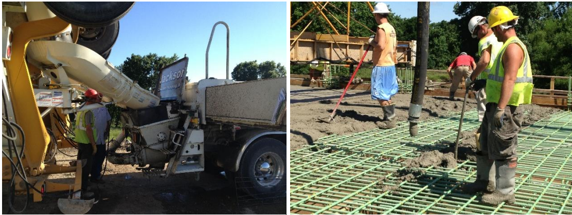
Figure 8. Concrete being discharged to a pump truck and then to the deck
