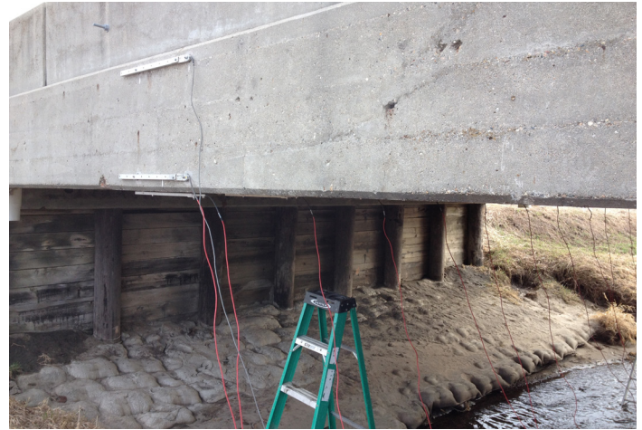
Strain gauges installed on concrete slab bridge
