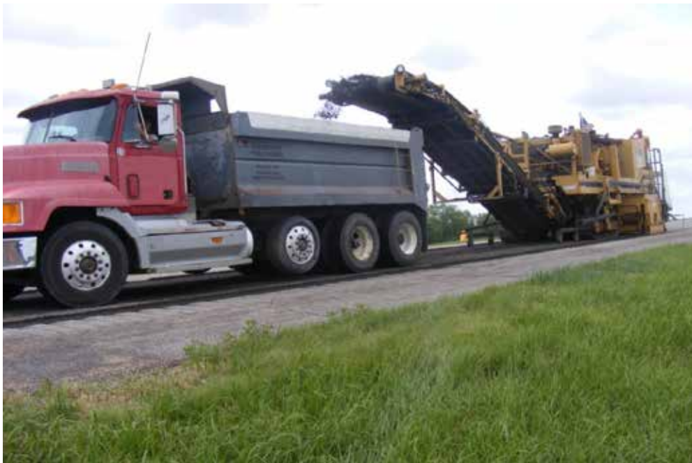
Figure 1.2: Pavement Milling
