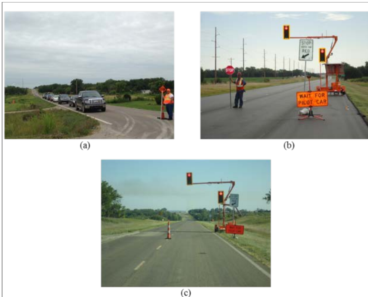
Figure 4.2: Three Study Conditions: (a) Flagger Only; (b) PTS with a Flagger; (c) PTS without a Flagger
